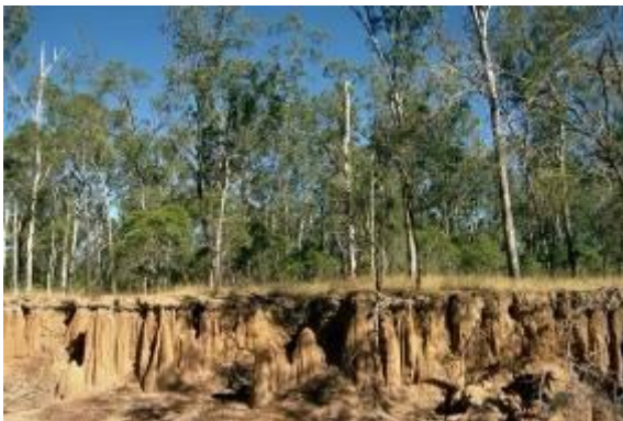
Photograph 47. Severe gully erosion on Ulogie soil due to the highly dispersive subsoil
