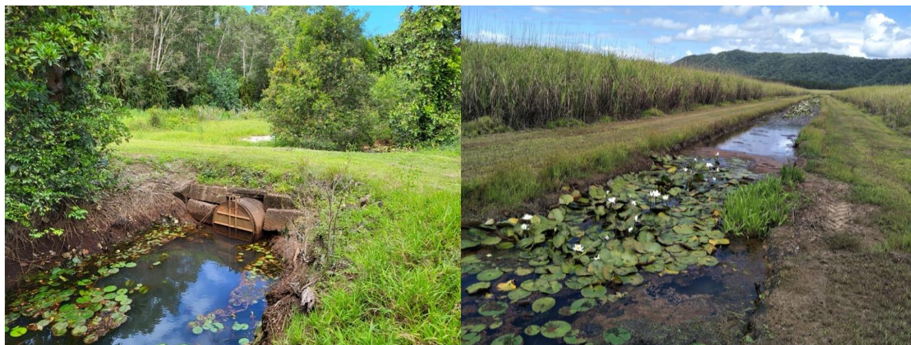
Figure 25: Example of a one-way tidal gate at Site 1 (left) and drain (right) on the site with a range of aquatic freshwater invasive plants and some natives.
