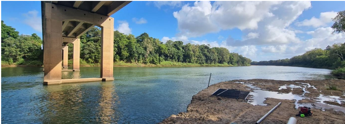
Figure 38. Herbert River at John Row Bridge monitoring infrastructure (looking upstream).
