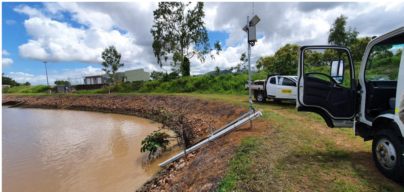
Figure 2: Micro-site infrastructure from Burdekin River at Tom Fenwick Pump Station. The site was installed within the retention dam fed directly from water pumped from the adjacent Burdekin River. From this point, water is pumped into an artificial irrigation network.
