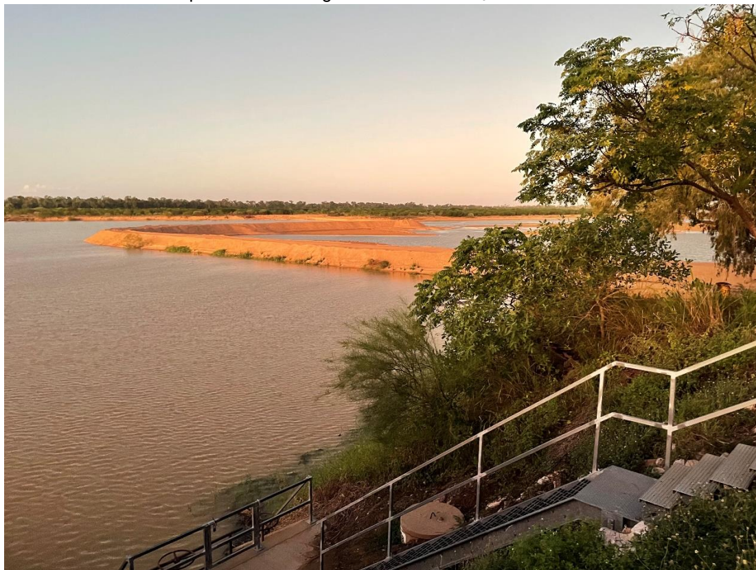
Figure 21: Burdekin River at Down River Pump Station monitoring site is co-located with Lower Burdekin Water pump infrastructure. Photo is looking downstream showing the sand dam has been constructed.
