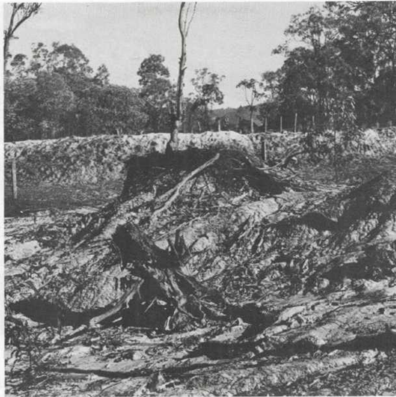
Gully erosion is a serious problem within a number of the mapping units in the study area. This photo shows gully erosion occurring on the Gatton Sandstone Mapping Unit.
