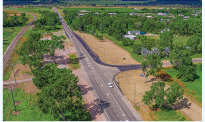
Alligator Creek Bridge to Alligator Creek Road intersection upgrade, south of Townsville (June 2021).
