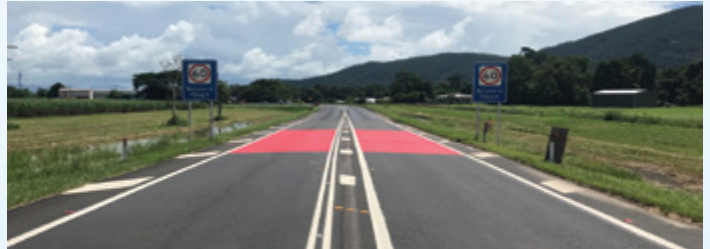
Township Entry Treatment approaching Tully, completed 2021.
