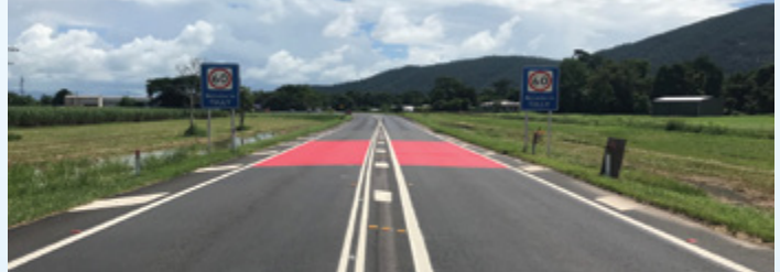
Township Entry Treatment approaching Tully, completed 2021.
