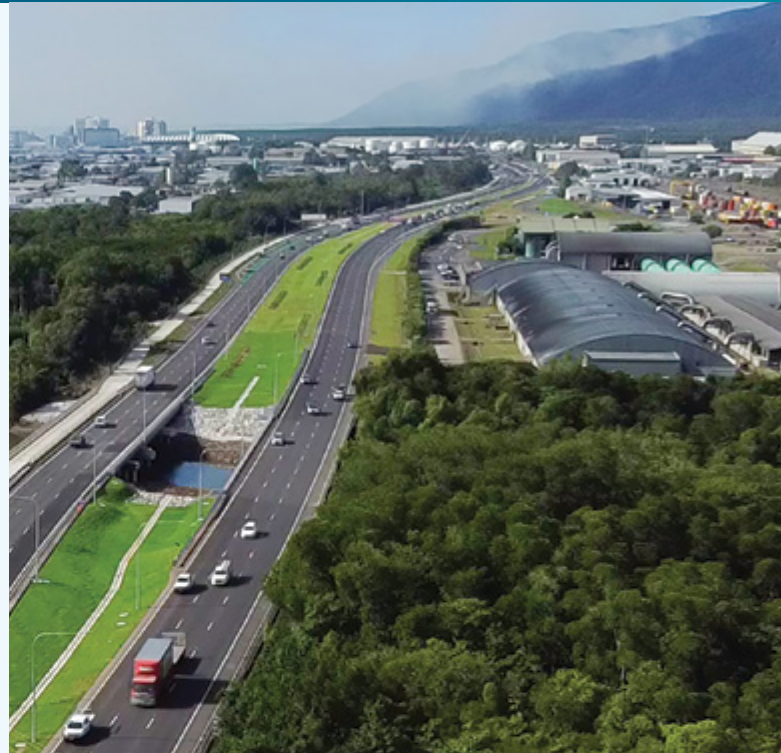
Cairns Southern Access Corridor (Stage 4), Kate Street to Aumuller Street, Peter Moss Bridge over Chinaman Creek (June 2021).
