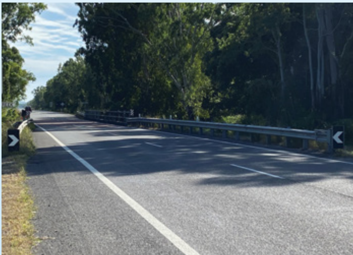
Palm Creek narrow bridge.
