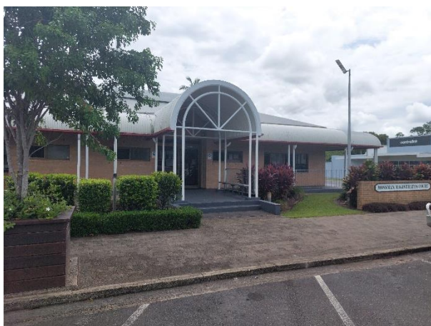
Figure K.3 Mossman courthouse
