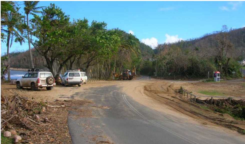
Photo 26. Beach sand washed some 20m inshore across Alexander Drive at Bingil Bay.
