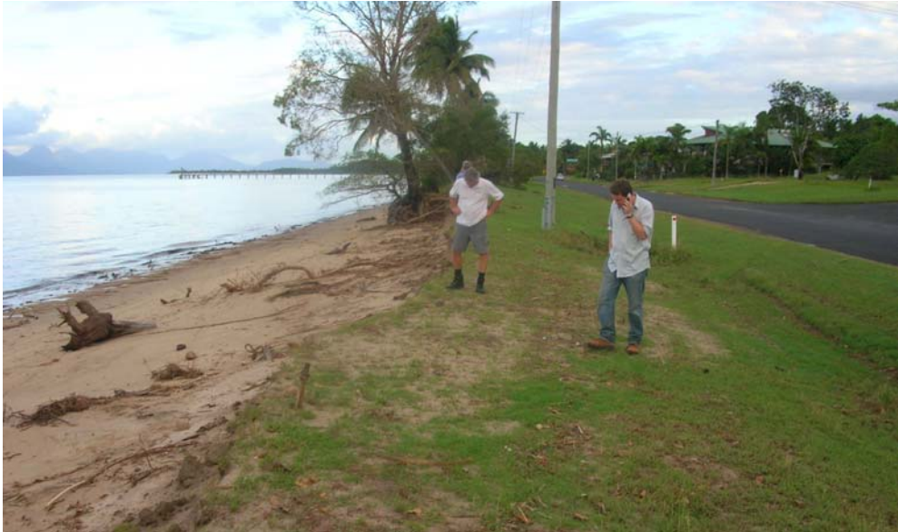
Photo 46. Debris line at Cardwell indicates slight overtopping of the dune.
