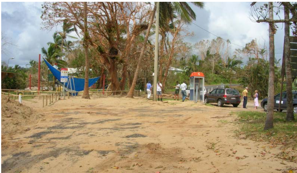
Photo 4. Beach sand washed across the park area at Flying Fish Point.
