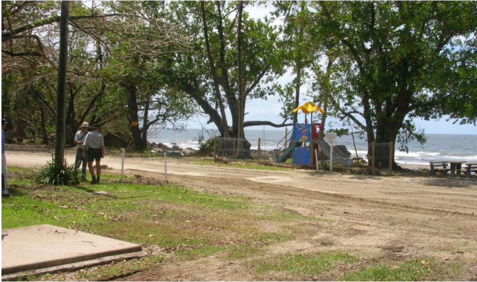
Photo 7. Debris line landward of pole at ETTY Bay.
