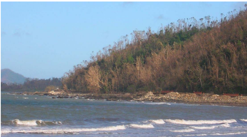
Photo 27. A rock wall protecting the road around Clump Mountain failed (south of Bingil Bay).
