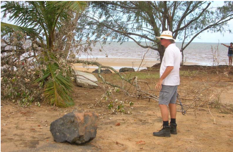
Photo 20. A concrete slab was moved from near the boat ramp by the storm tide. Also pictured is a boulder from the rock wall.
