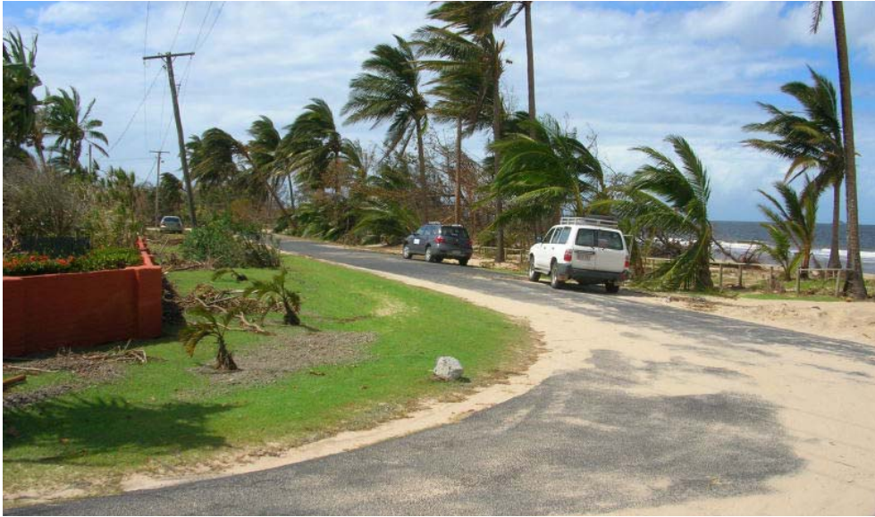
Photo 13. Debris lines along property boundaries at Cowley beach.
