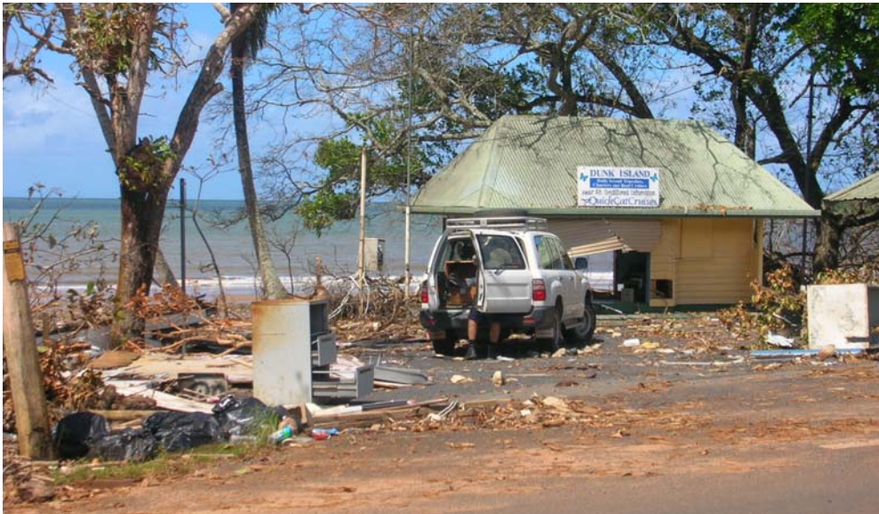
Photo 29. The storm tide caused structural damage to "Quick Cat Cruises" offices at Clump Point.
