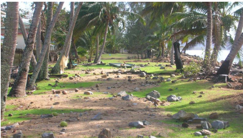
Photo 45. Sand and rocks washed inshore of the rock wall at Tully Heads by wave overtopping.
