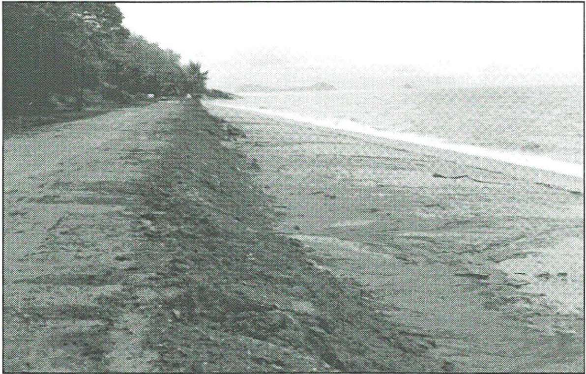
Trinity Beach (northern end). Erosion along this section of beach was caused by wave action and water run-off.
