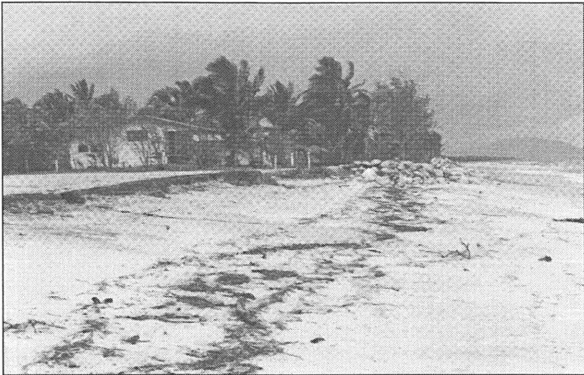
Tully Heads. Minor slumping of the rock wall was evident.
