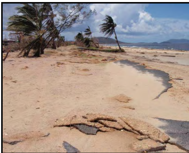
Photograph 27: Sand intrusion, vegetation damage and road destruction caused by TC Yasi at Tully Heads (Source: DSITIA)
