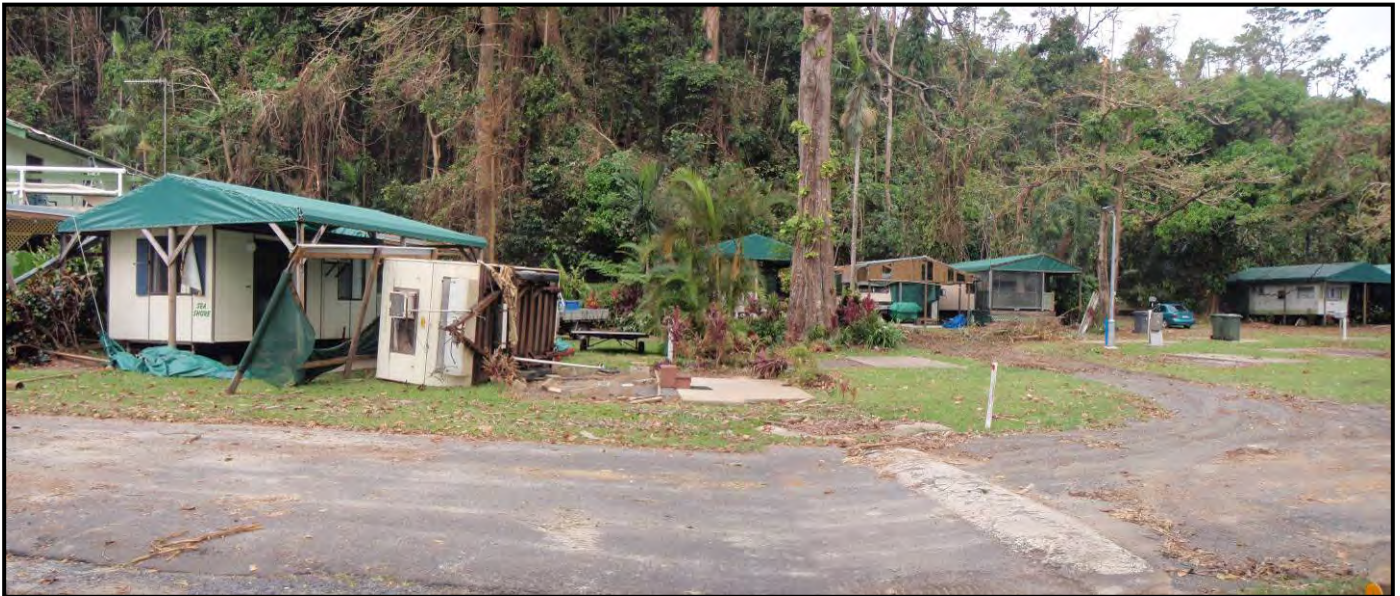
Photograph 7: Damage caused by TC Yasi at Etty Bay (Source: DSITIA)
