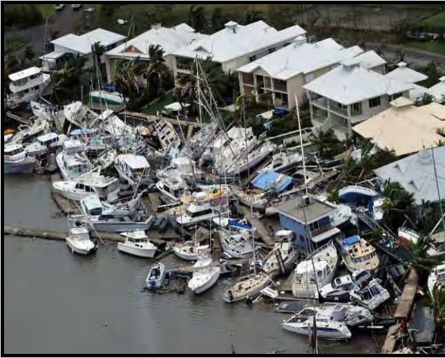
Photograph 30: Damage to Port Hinchinbrook Marina, Cardwell, caused by TC Yasi (Source: News Limited)
