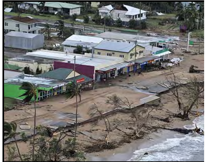
Photograph 31: Coastal erosion and damage to buildings and infrastructure at Cardwell following TC Yasi (Source: News Limited)
