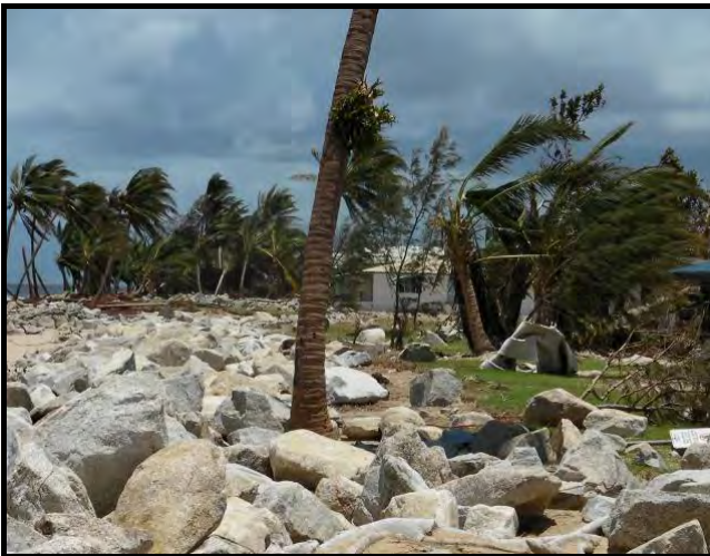
Photograph 22: Armour rocks from the seawall washed up by storm surge and increased wave energy during TC Yasi (Source: DSITIA)
