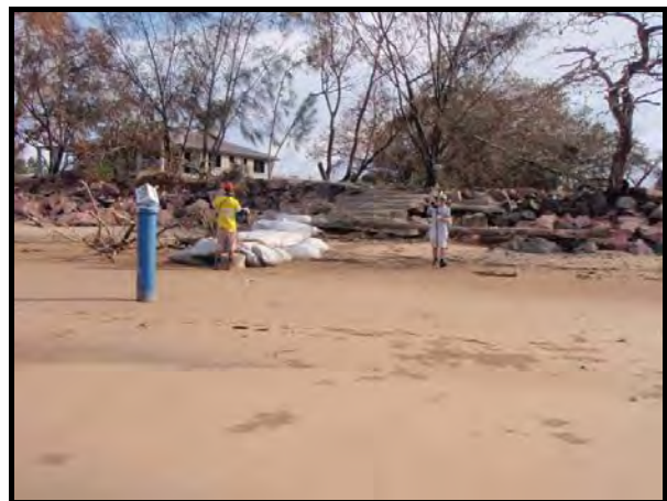
Photograph 34: Damage to Lucinda foreshore (Source: DSITIA)
