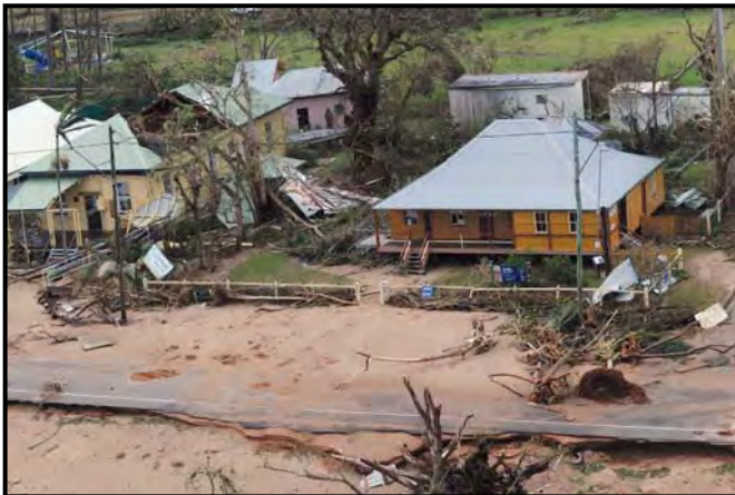
Photograph 40: The 5.33 metre storm surge during TC Yasi, 3 February 2011, damaged the Cardwell esplanade and deposited sand and debris above HAT (Source: News Limited).
