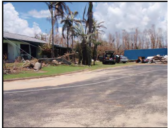
Photograph 23: Building damage and relocation of shipping container during TC Yasi (Source: DSITIA)
