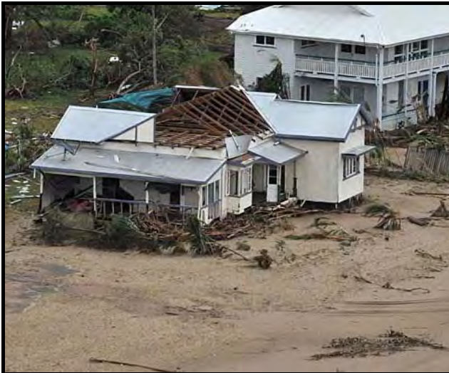
Photograph 28: Damage to houses at Cardwell caused by TC Yasi (Source: News Limited)
