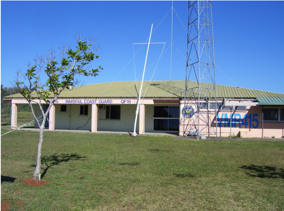
Coast Guard building at Mourilyan Harbour, the flagpole has been structurally damaged by the cyclone, notice the tree in the foreground has also been damaged and is at a similar angle to the flagpole
