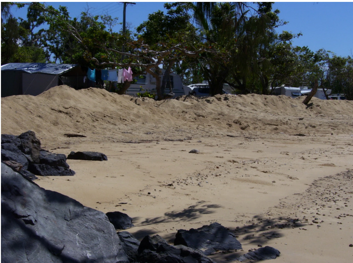
Sand dumped along the vegetation line in front of the caravan park
