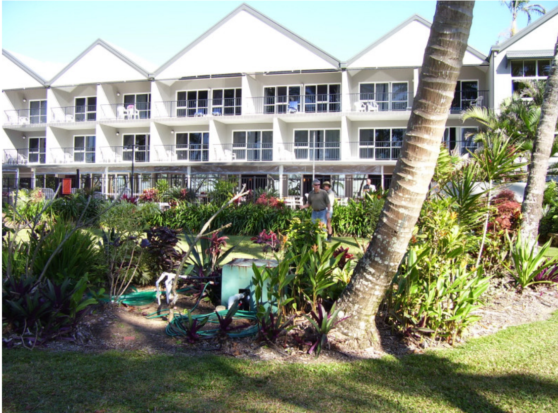
Location of inundation line in front of the pool at Castaways (when men are standing)
