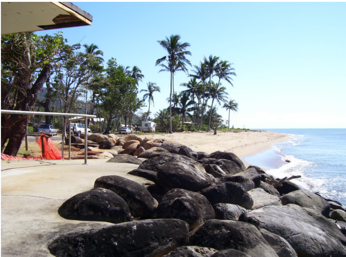
Looking north from in front of the toilet block at the southern end of Flying Fish Point
