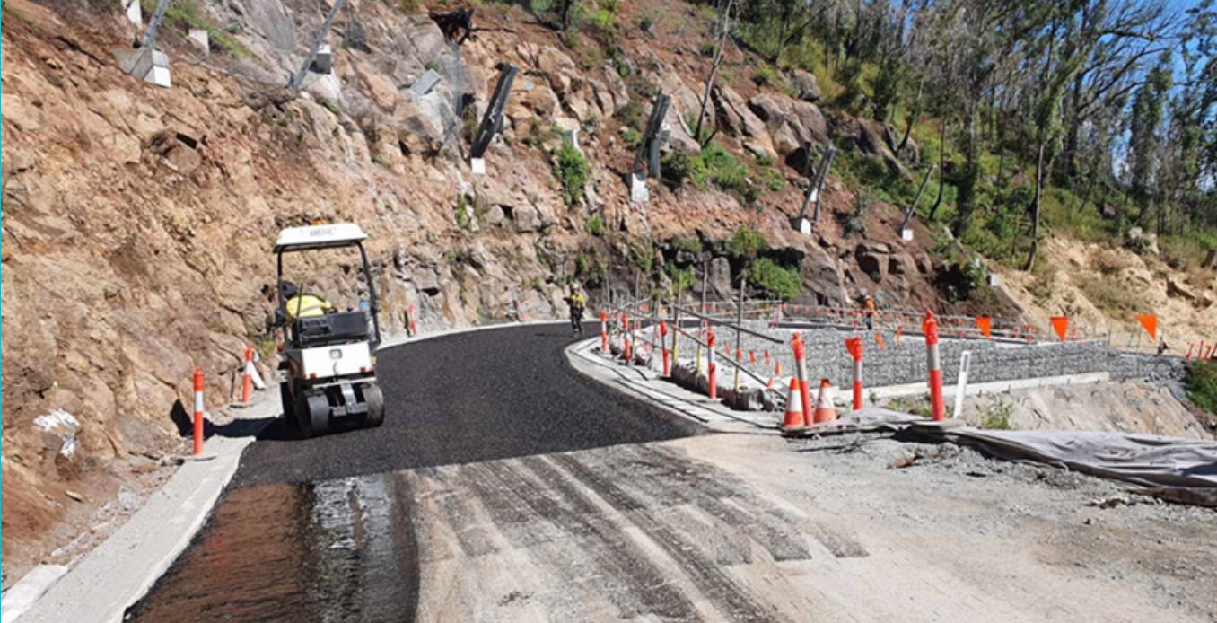
Restoration progress along Binna Burra Road, May 2020
