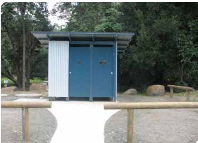
Roadside rest area toilet block
