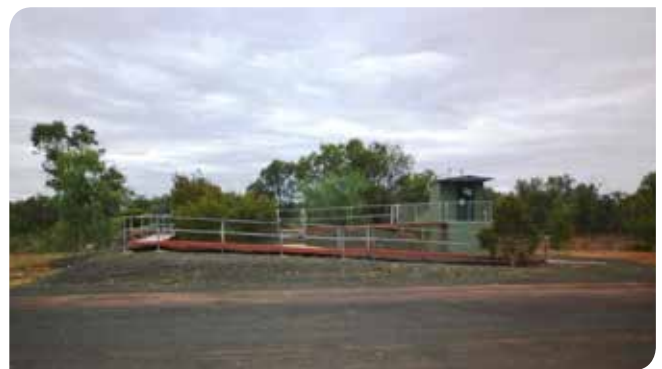
Natural Sciences Loop—roadside rest area toilet and all abilities access ramp
