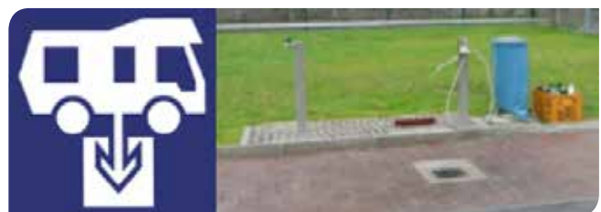
Signage and in-ground dump points
