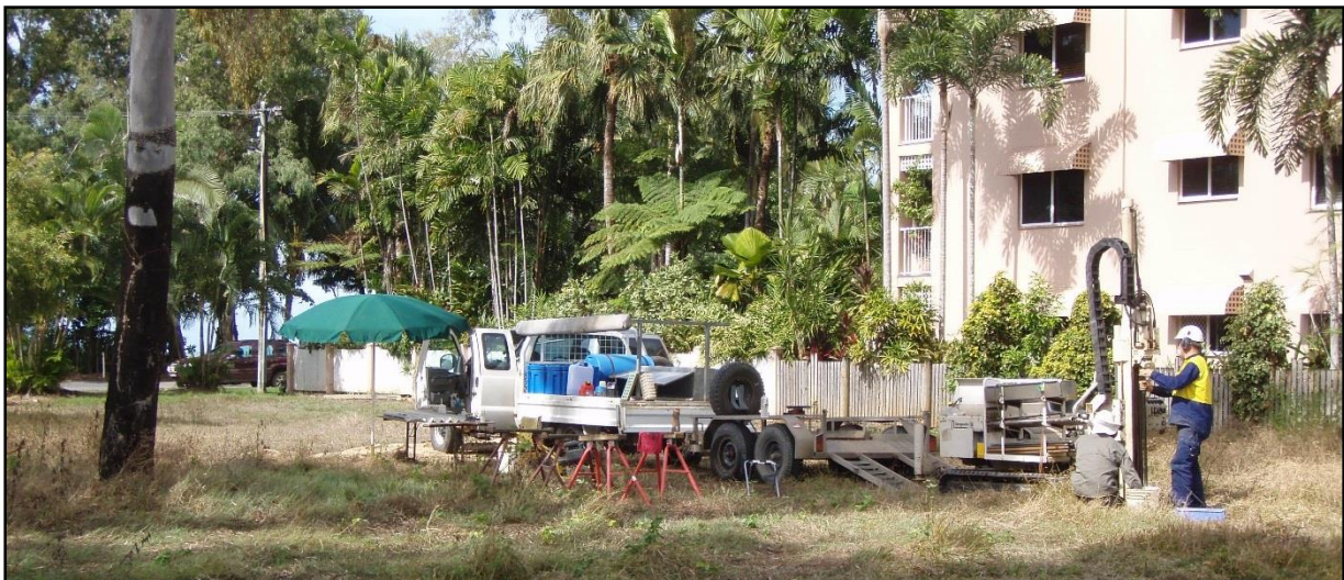
Plate 3. Site 237, Location: Clifton Beach, Map unit: S3, LiDAR elevation: 3.6m AHD, PASS depth: 3.4m, PASS elevation 0.2m AHD.
