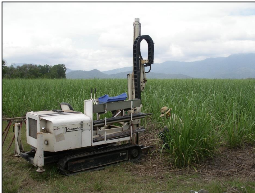
Plate 1. Geoprobe model 54DT track-mounted coring machine
