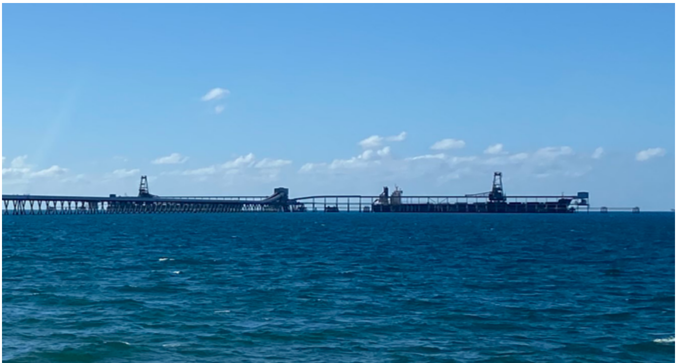
Bulk vessels at the Port of Abbot Point. Source: TMR
