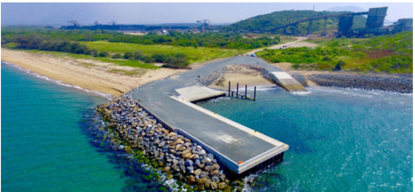
Abbot Point Marine Offloading Facility. Source: NQBP
