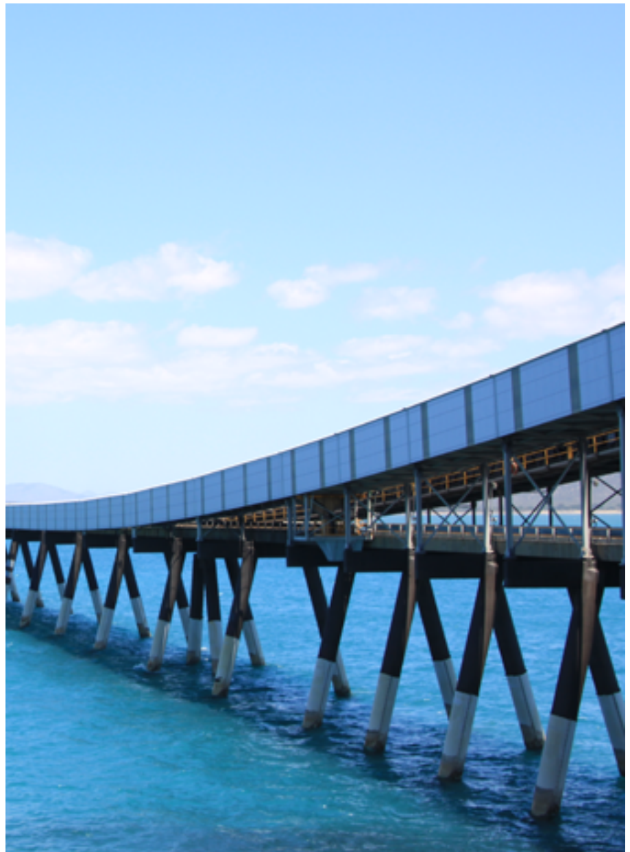
Berth at the Port of Abbot Point. Source: NQBP
