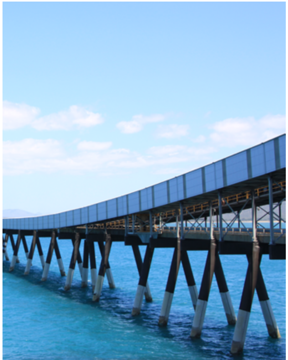
Berth at the Port of Abbot Point. Source: NQBP
