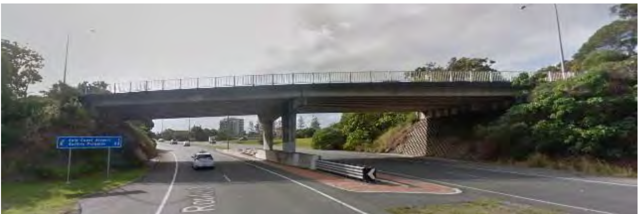
Figure 3-33 Bridge street view (Source: google streetview)
