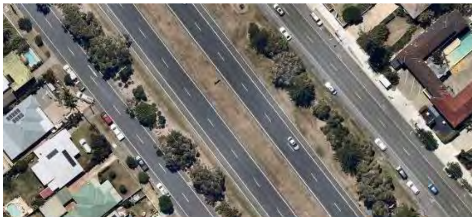
Figure 3-3 Gold Coast Highway (Bilinga and Airport) typical carriageway (Image source: Metromap 2020)
