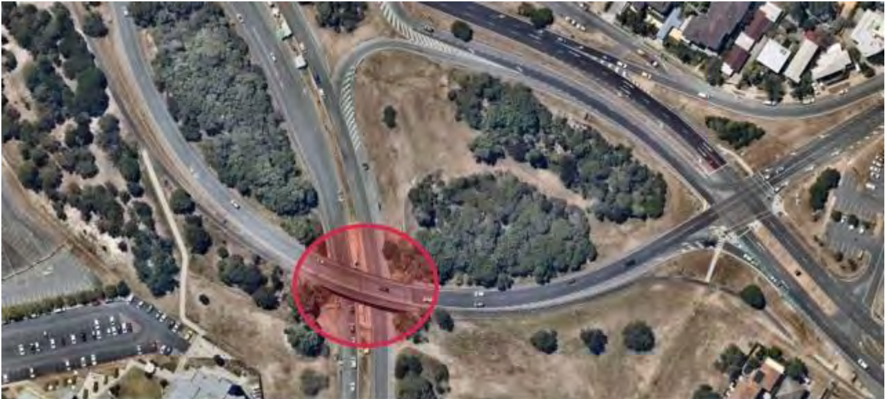
Figure 3-32 Bridge location on interchange (Image source: metromap, 2019)
