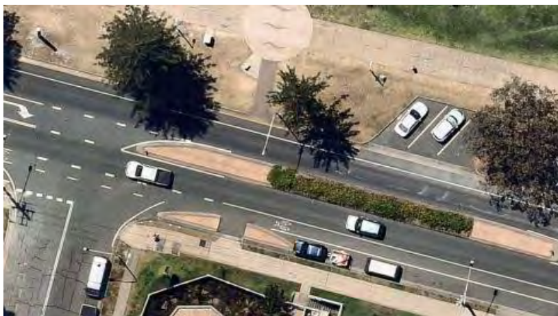
Figure 3-5 Musgrave Street (Kirra) typical carriageway (Image source: Metromap 2020)
