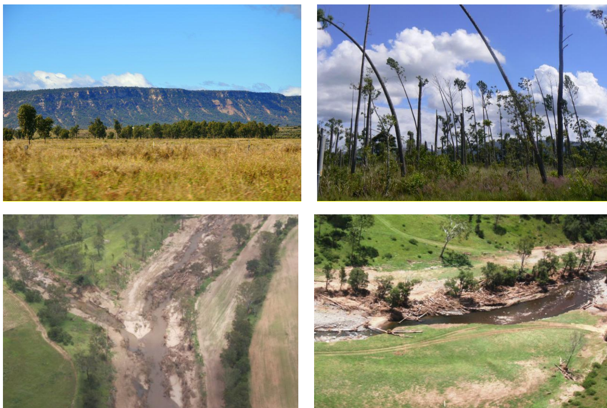
Figure 6: Example of landslips near Carnarvon Gorge (top left), Cyclone Yasi damage in pine forest near Cardwell (top right) and flood damage in South East Queensland (lower images).
