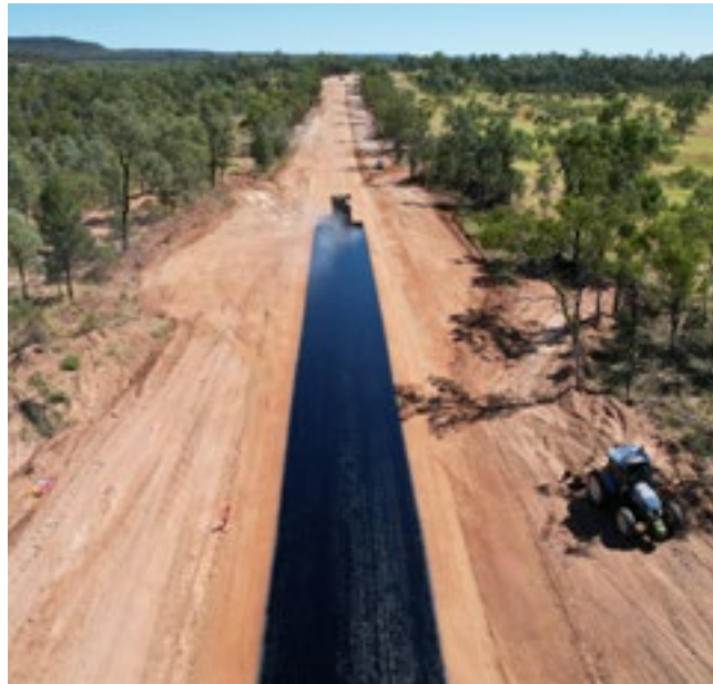
▲ Sealing of Mt Tabor Road, Murweh Shire Council
