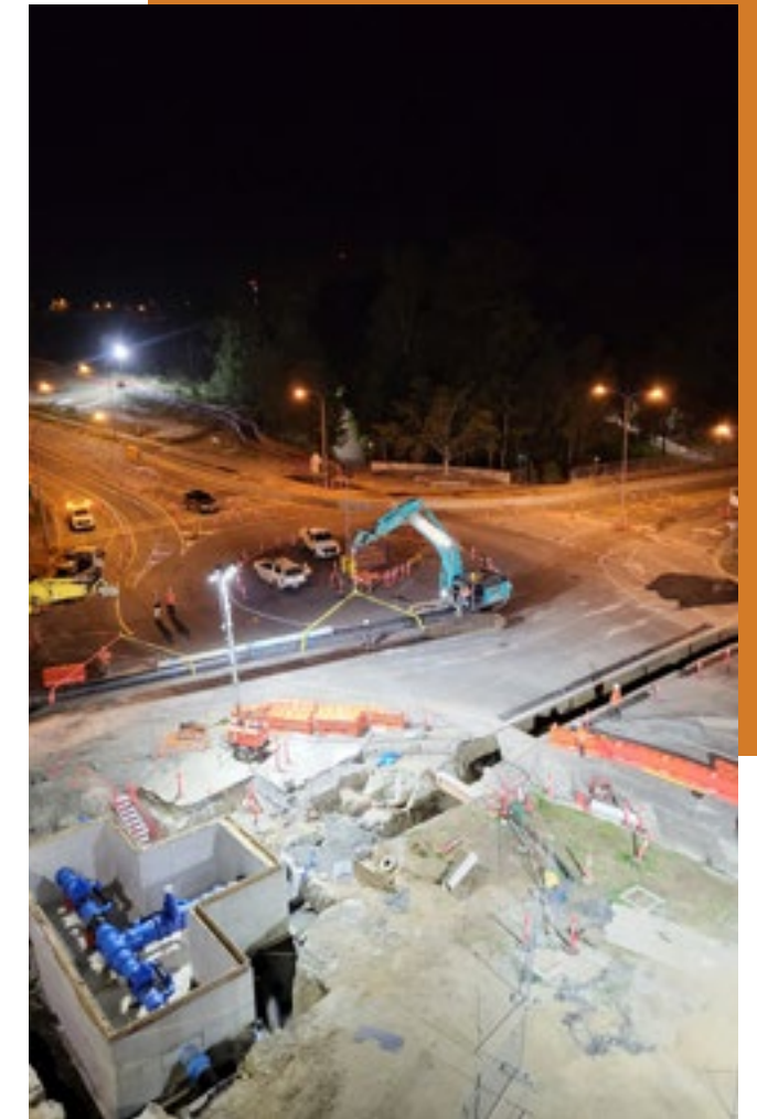
Urban utilities pit works at Exit 32 Centenary Motorway, Ipswich City Council
