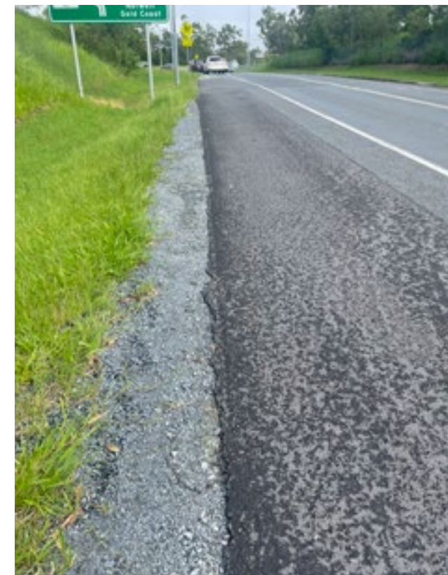
Tillyroen Road, Gold Coast City Council - post construction
