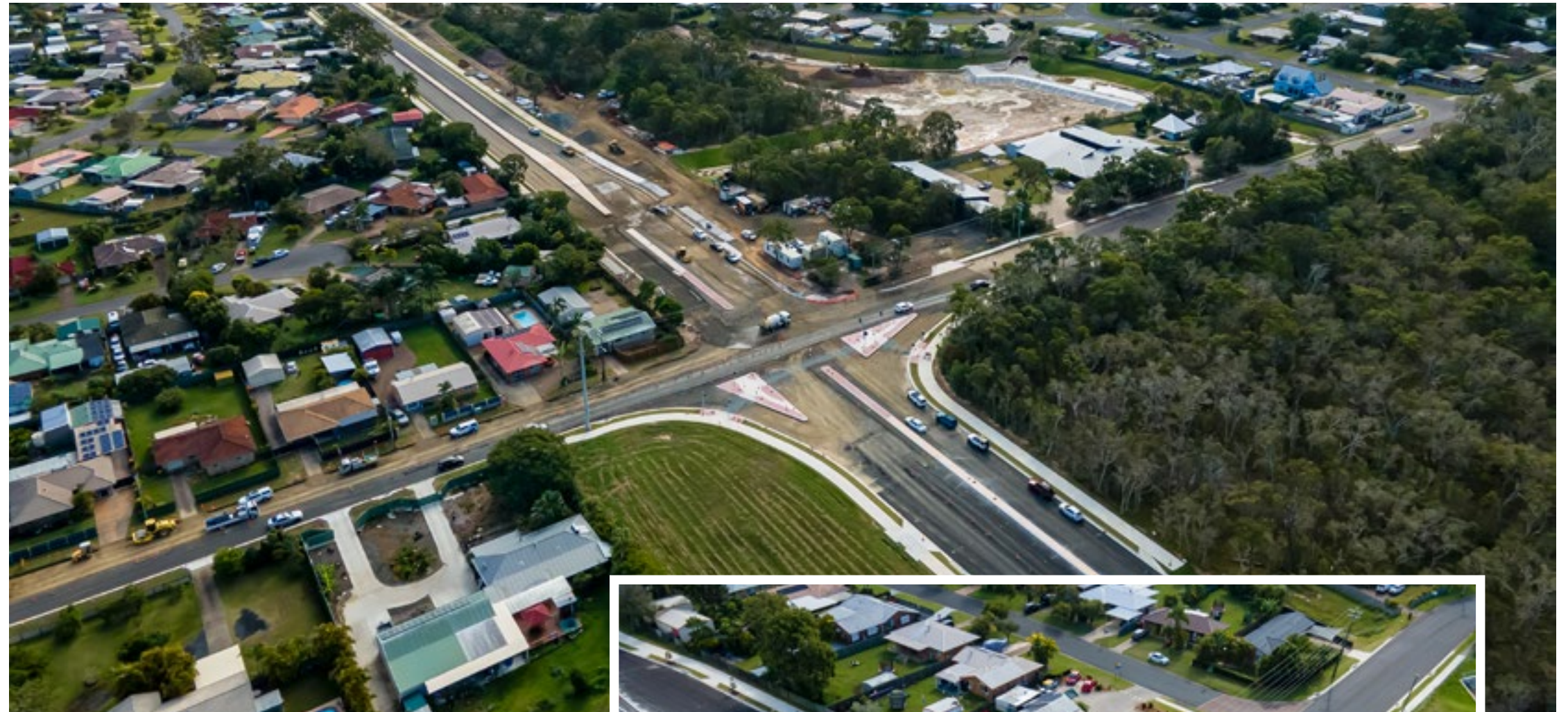
Aerial view of Boundary Road, Fraser Coast Regional Council - under construction
