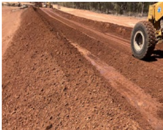
Jobs Gate Road, Paroo Shire Council - mixing of gravel prior to pavement
