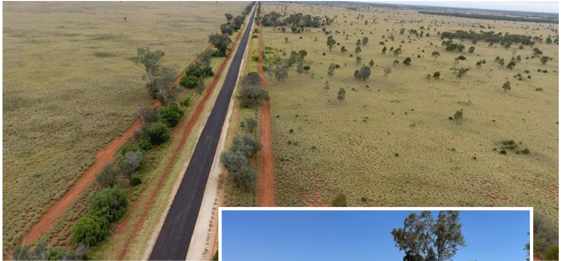
▲ Jakelwar-Goodooga Road North, Balonne Shire Council - completed
