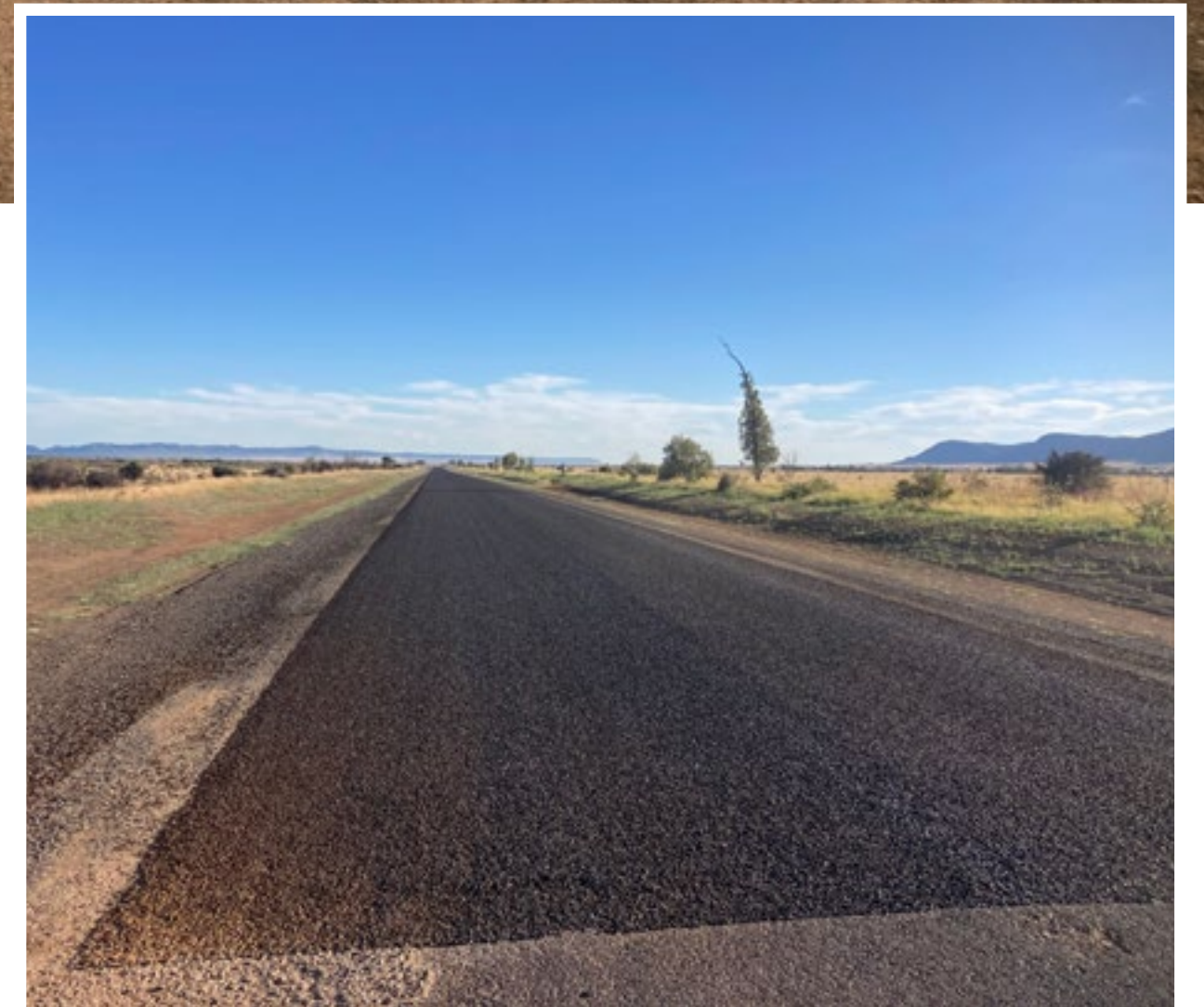
▲ Arcadia Valley Road, Central Highlands Regional Council after sealing
