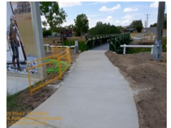
New pavement upgrade on Scottville Road, Whitsunday Regional Council
