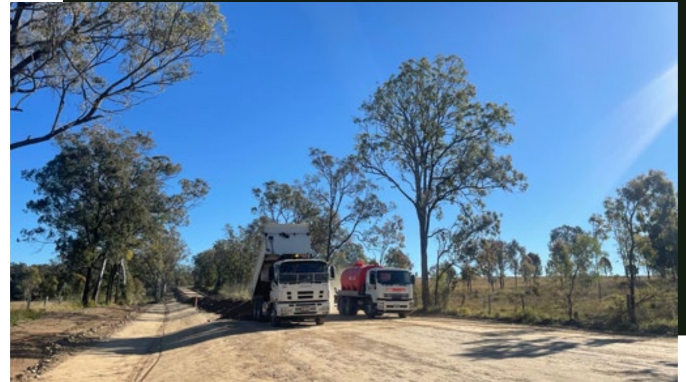
The upgrade of Maidenwell-Bunya Mountain Road, South Burnett Regional Council
