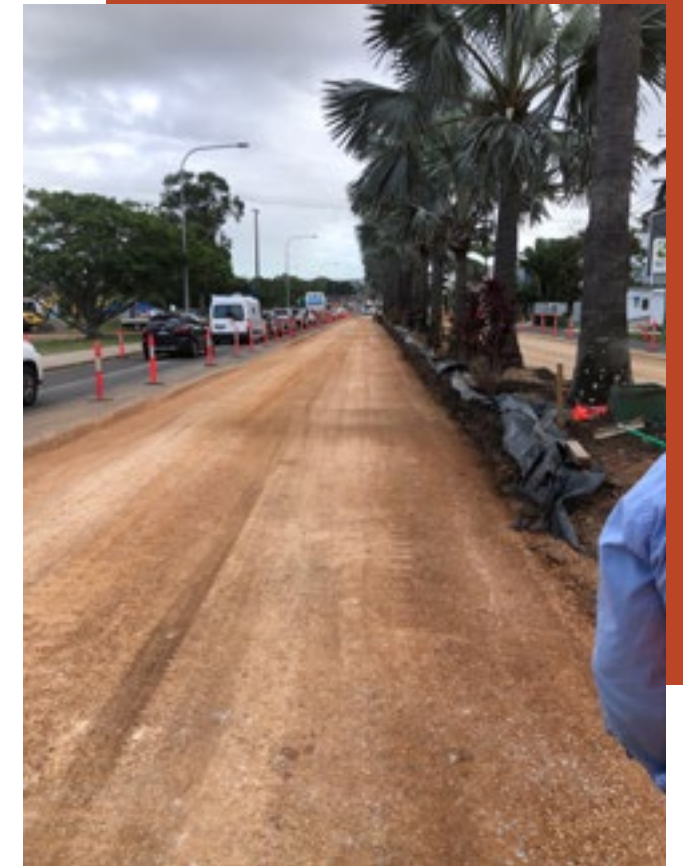
▲ Glenlyon Street, Gladstone Regional Council during construction
