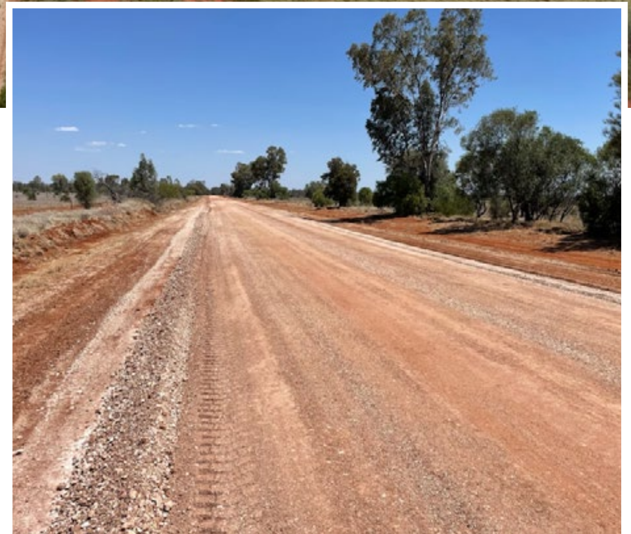
▲ Jakelwar-Goodooga Road North, Balonne Shire Council - during upgrade
