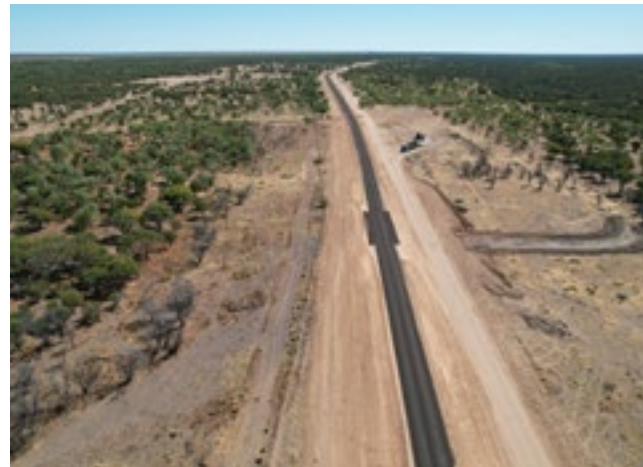
Taldora Road, McKinlay Shire Council - completed
