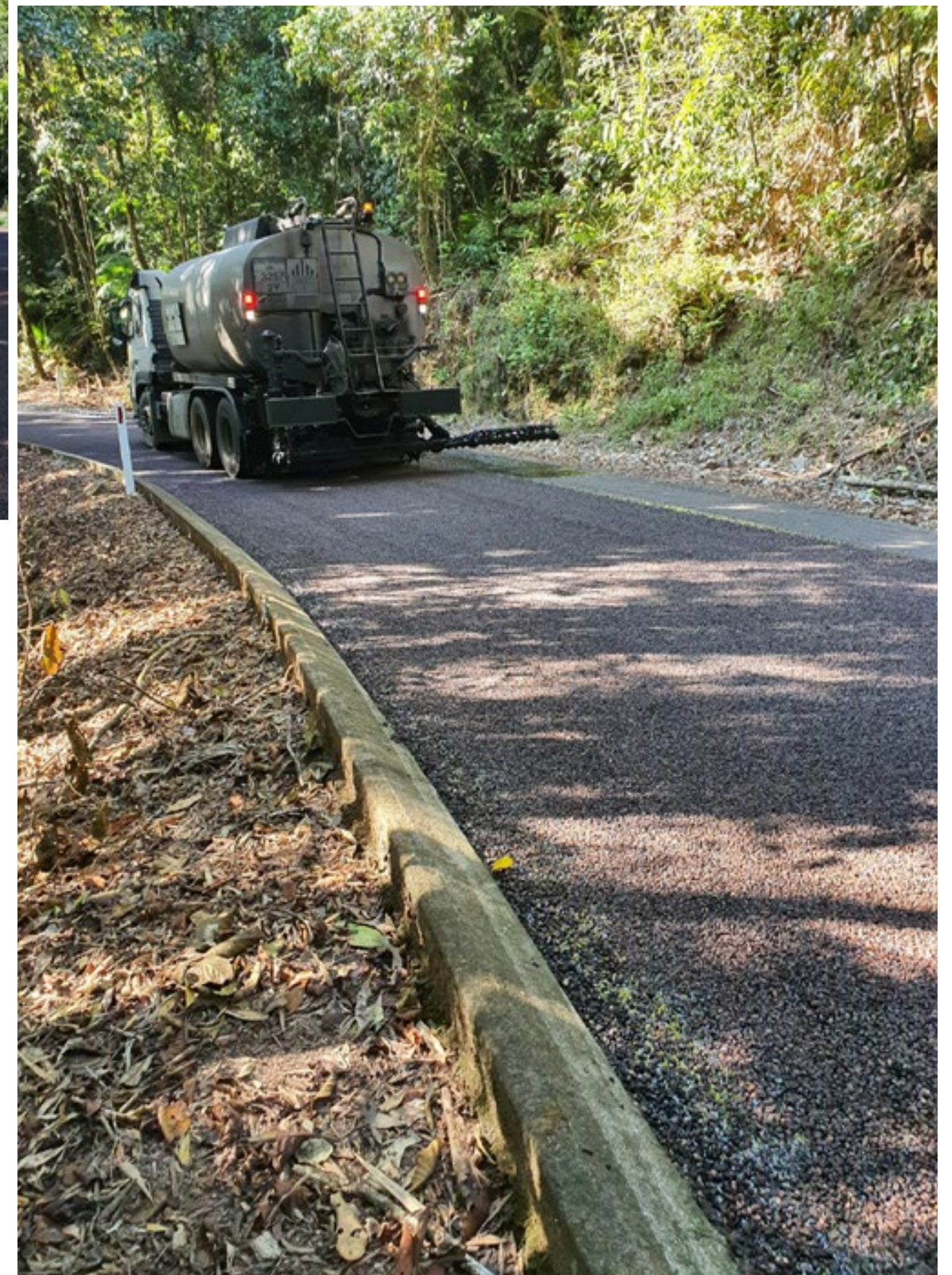
Sealing Wallaman Falls Road, Hinchinbrook Shire Council
