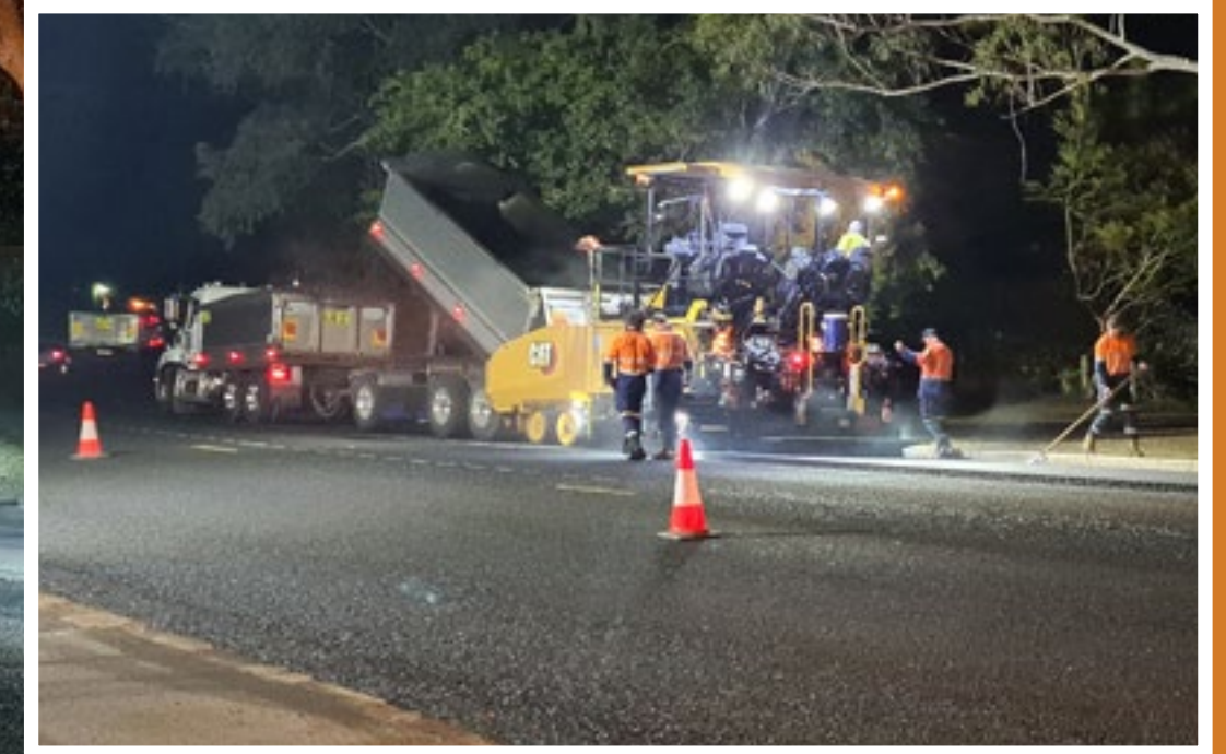
Butler Street, Noosa Shire Council - seal during construction ▶
