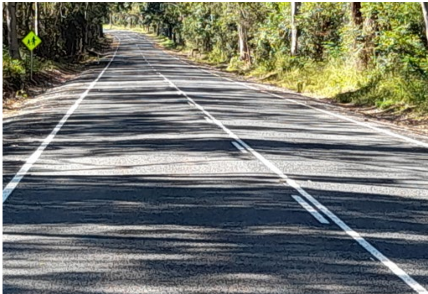
▼ Mt Tabor Road, Murweh Shire Council - completed
