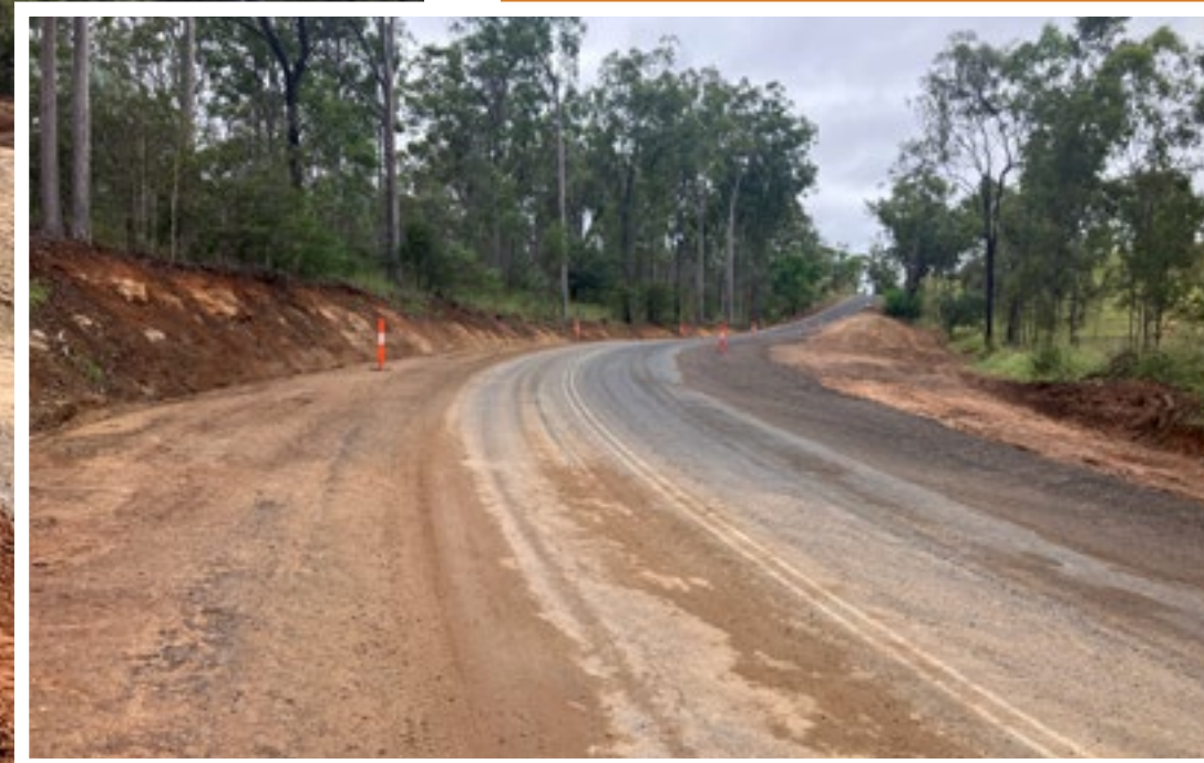
◀ Woodlands Road, Lockyer Valley Regional Council - during construction
