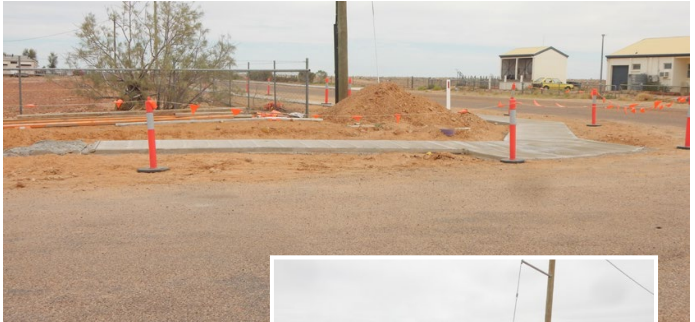
▲ Birdsville footpath, Diamantina Shire Council - installation
