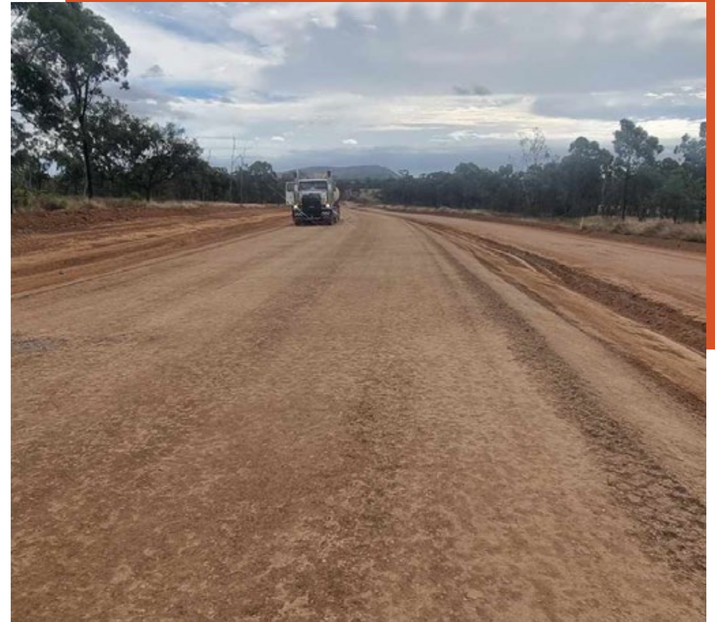
During construction on Dotswood Road, Charters Towers Regional Council
