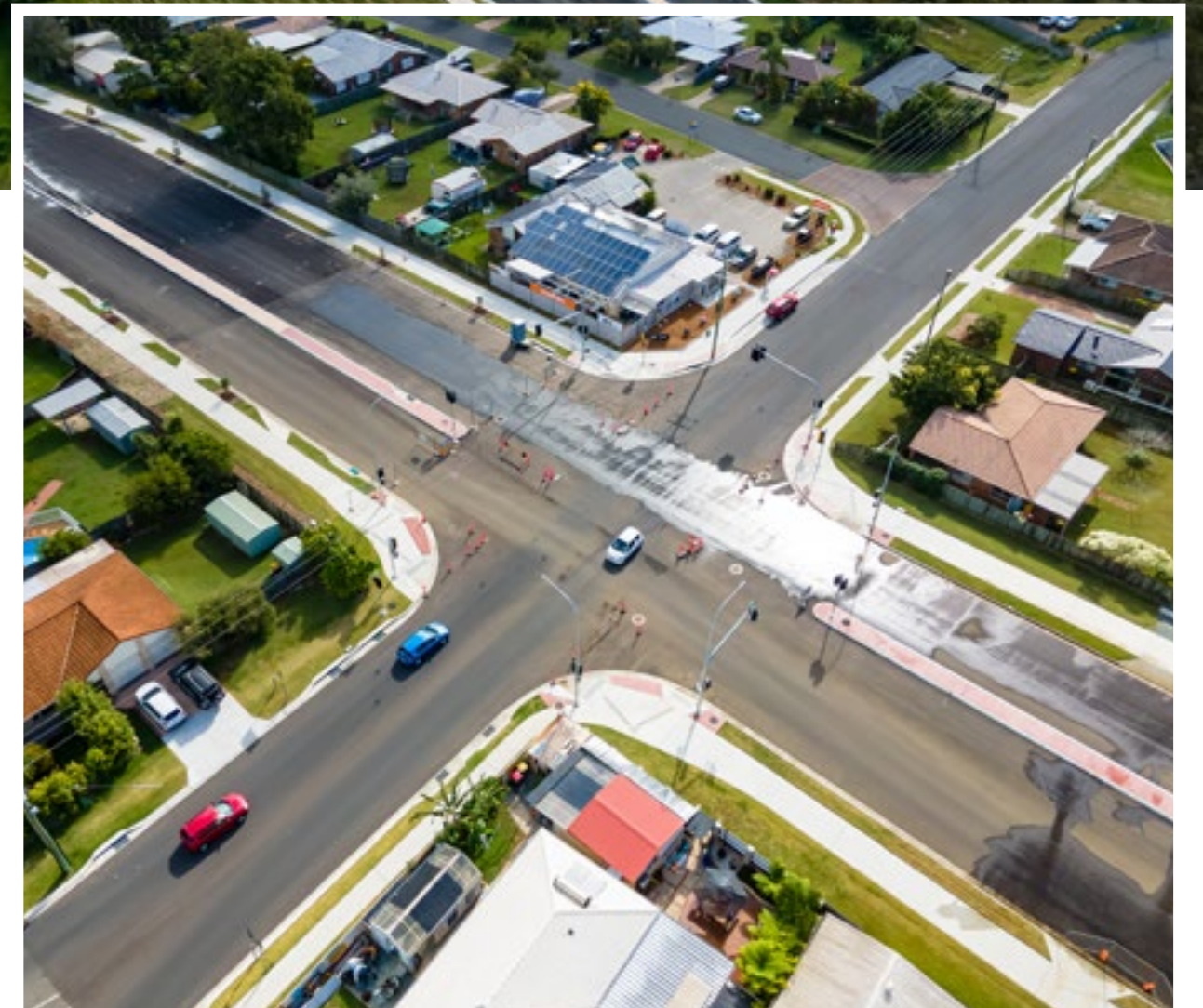
Boundary Road Extension Project, Fraser Coast Regional Council
