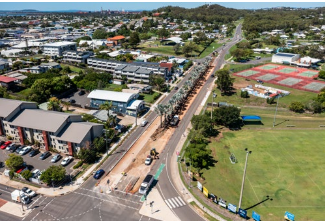
▲ Glenlyon Street, Gladstone Regional Council construction phase
