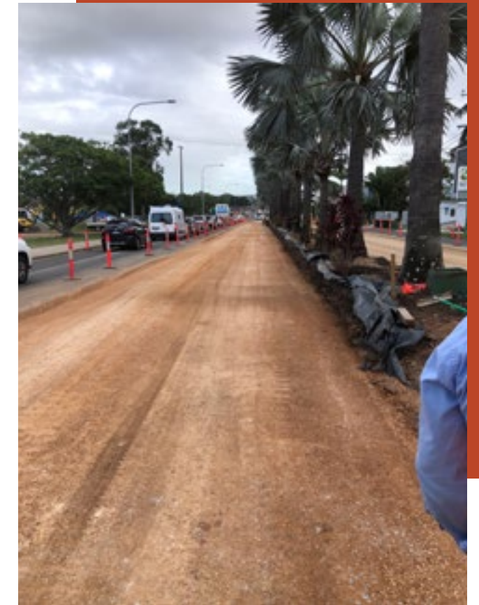
▲ Glenlyon Street, Gladstone Regional Council during construction
