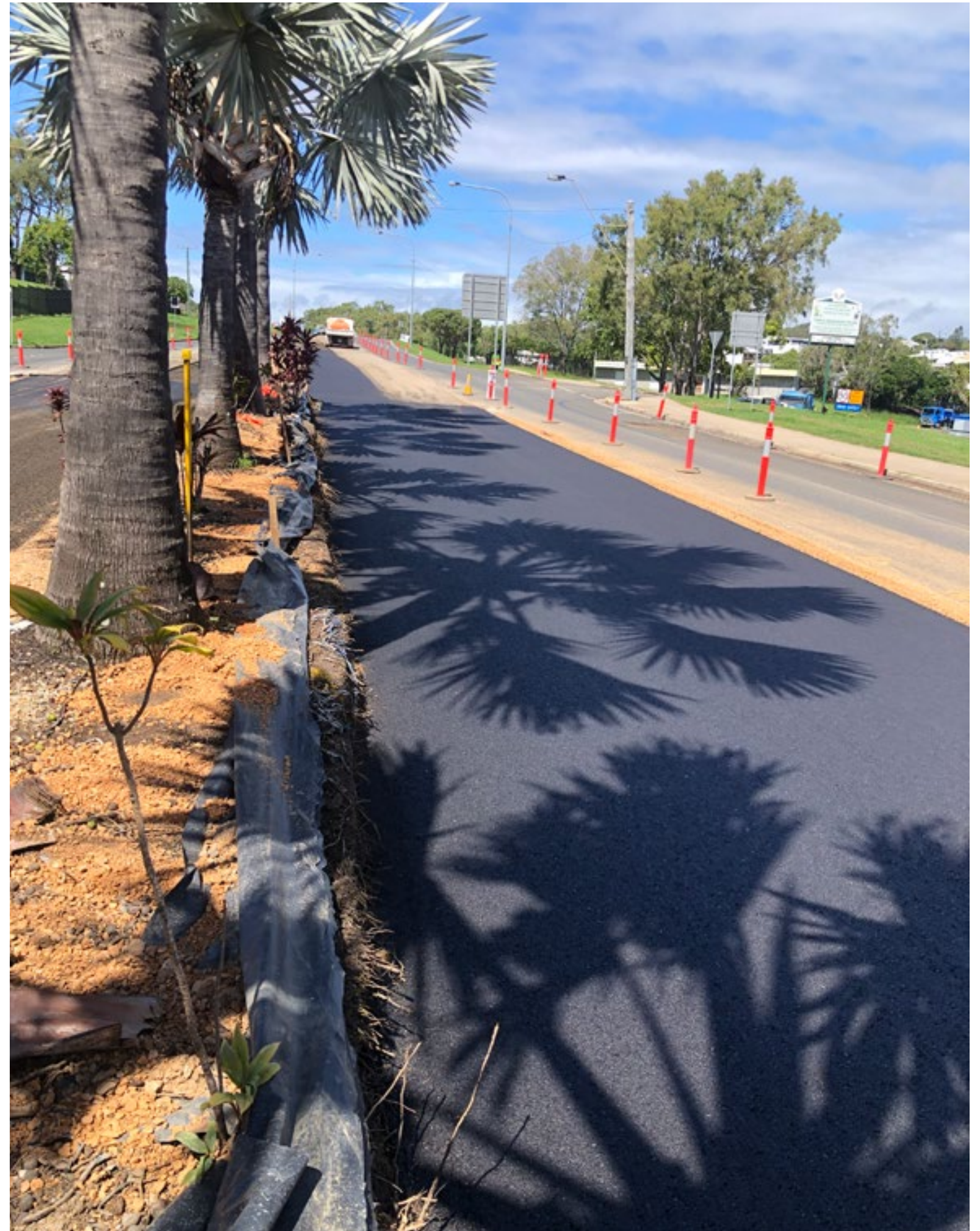
Glenlyon Street, Gladstone Regional Council - northbound lane
