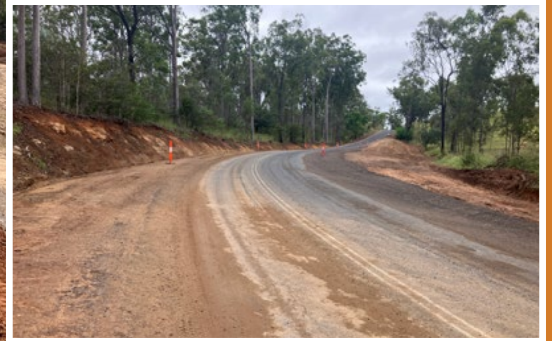
◀ Woodlands Road, Lockyer Valley Regional Council - during construction
