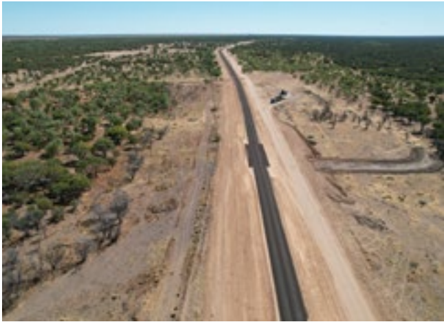
Taldora Road, McKinlay Shire Council - completed
