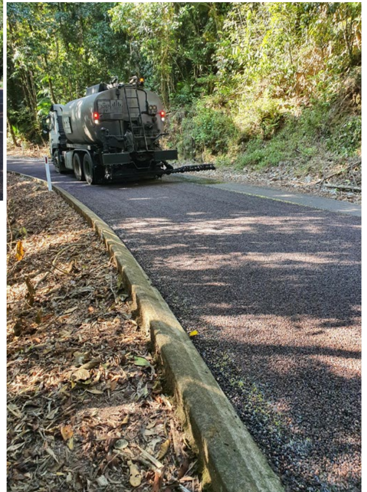
Sealing Wallaman Falls Road, Hinchinbrook Shire Council
