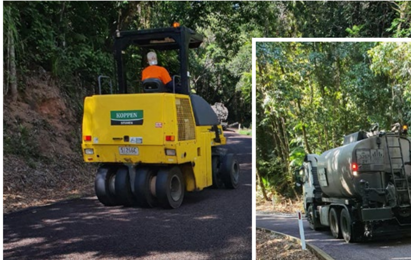
▲ Wallaman Falls Road, Hinchinbrook Shire Council - seal during construction
