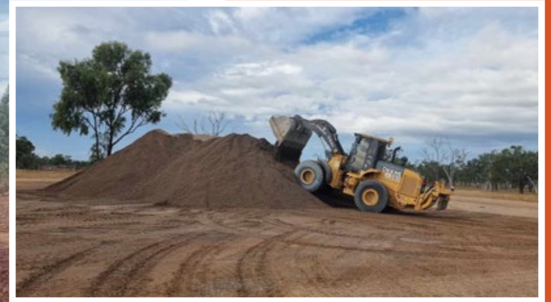
▲ Dotswood Road, Charters Towers Regional Council - loader during construction
