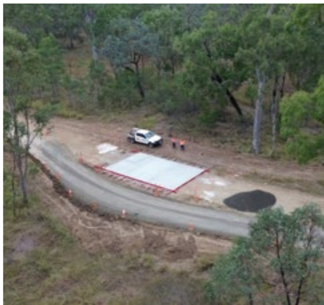
Aerial view of Harsants Road, Banana Shire Council during construction
