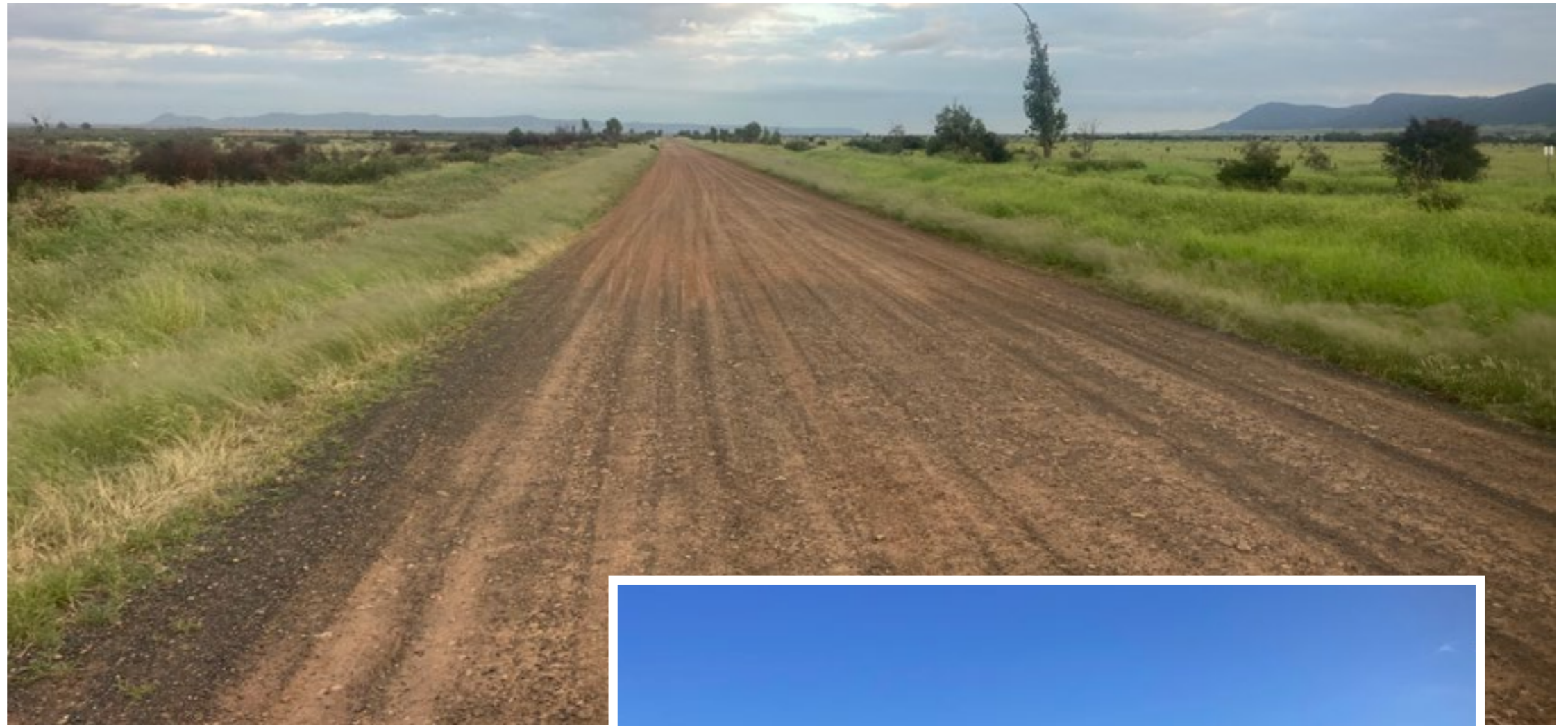
▲ Arcadia Valley Road. Central Highlands Regional Council pre-construction
