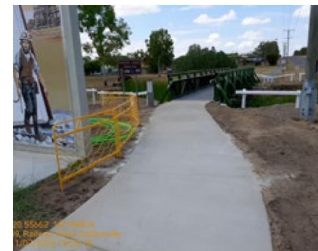
New pavement upgrade on Scottville Road, Whitsunday Regional Council
