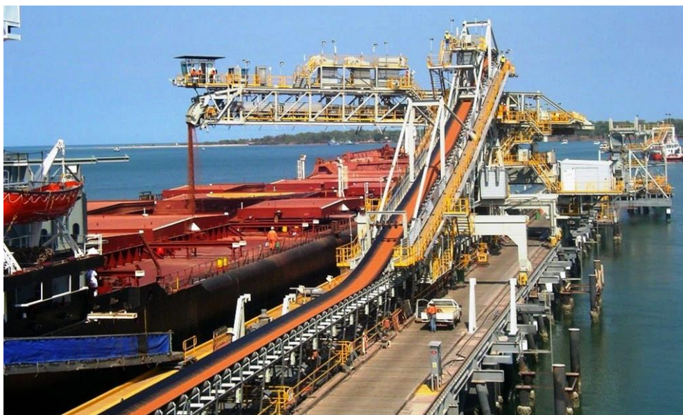
Figure 1 Ship loader at Weipa (courtesy NQBP)
