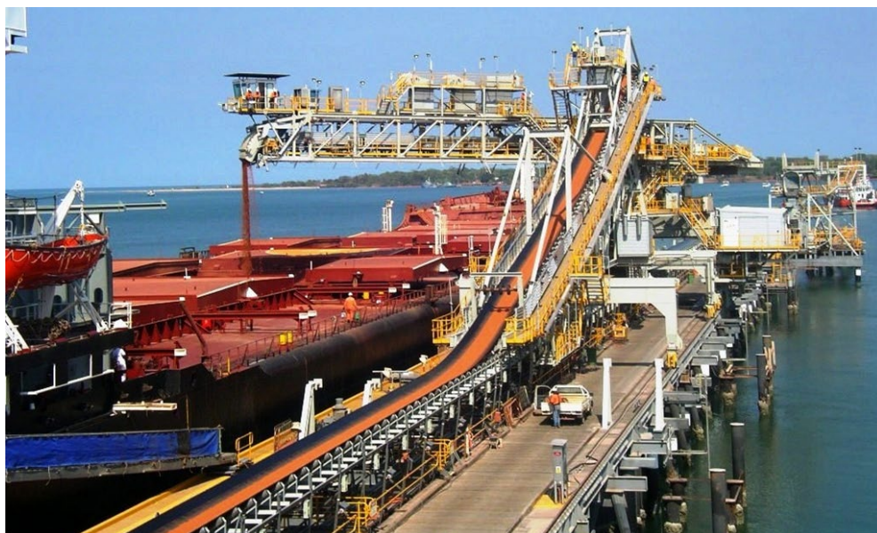
Figure 1 Ship loader at Weipa (courtesy NQBP)
