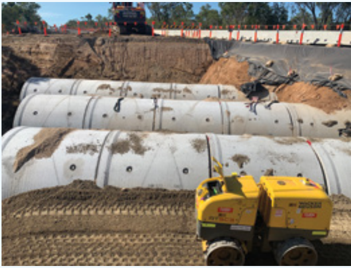
Culvert installation at Ten Mile Creek to Yeates Creek project (December 2021).
