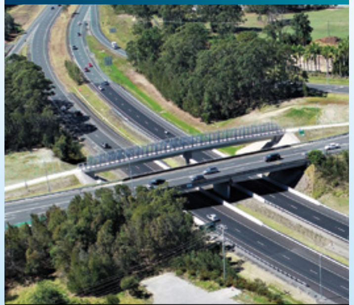
Sippy Downs interchange featuring new active transport bridge.
