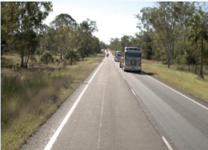
Single carriage section of the Bruce Highway between Gin Gin and Benaraby (2021).
