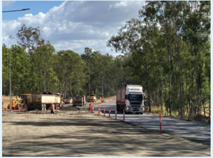
Maryborough to Gin Gin, Apple Tree Creek pavement widening (May 2021).
