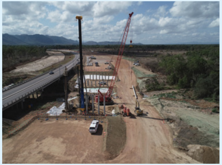
Townsville Ring Road Stage 5, Riverway Drive to Little Bohle River Bridge piling works (October 2021).
