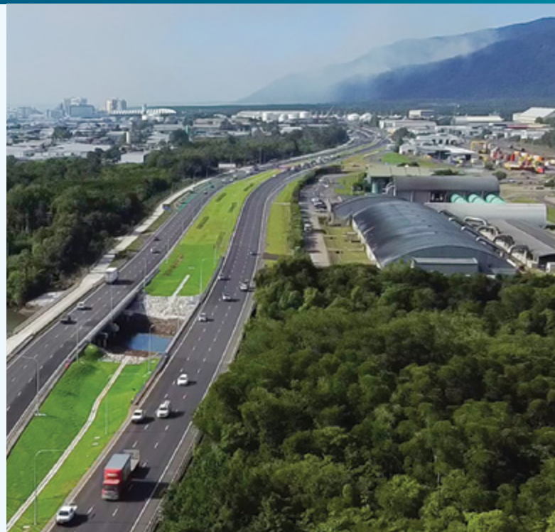
Cairns Southern Access Corridor (Stage 4), Kate Street to Aumuller Street, Peter Moss Bridge over Chinaman Creek (June 2021).
