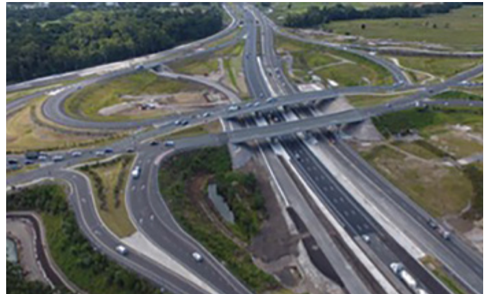
Caloundra Road to Sunshine Motorway, Diverging Diamond Interchange (April 2021).
