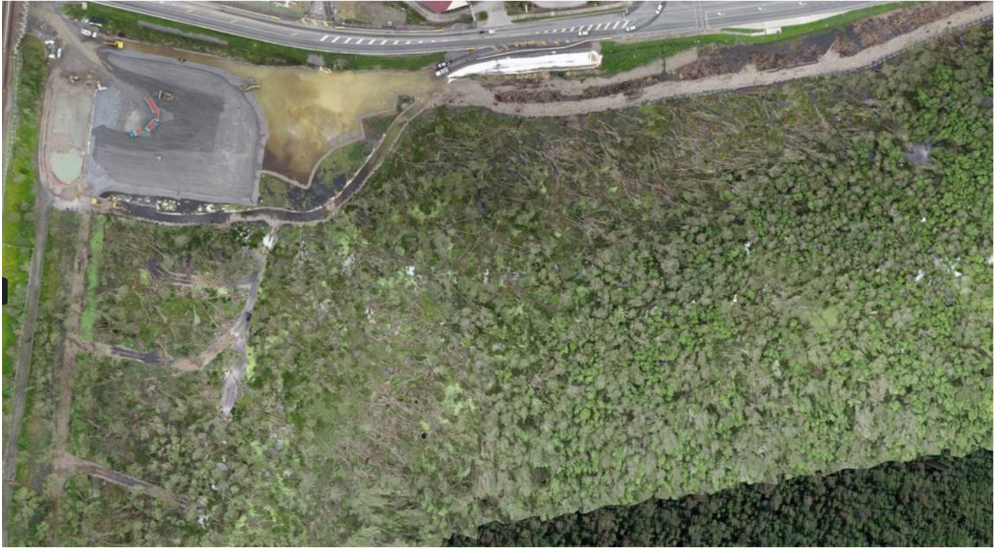
Figure 2: Aerial view of Helensvale Road after storm
