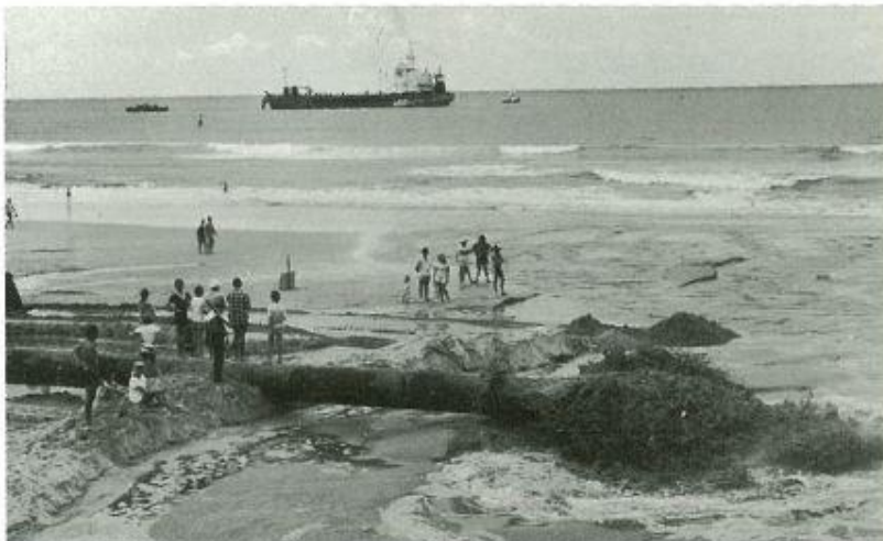
The dredge Vlaanderen XX is shown here pumping sand onto Burleigh Beach. The dredge was under contract to the Gold Coast City Council and discharged 200 000 m 3 of sand onto the beach and a further 100 000 m 3 in the nearshore zone at Burleigh.
