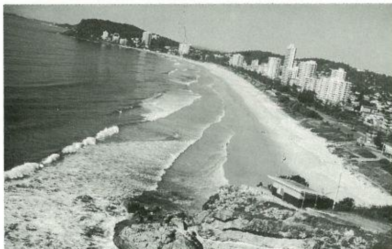
View of Burleigh Heads Beach looking south towards Burleigh Headland following the recent beach nourishment works. South Nobby Headland is in the foreground while the public park along the foreshore can also be seen.
