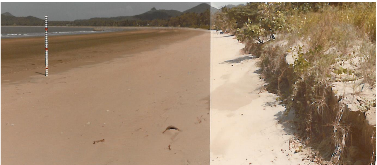
Figure 119 Seaforth Beach South February 1984 (Looking South)
