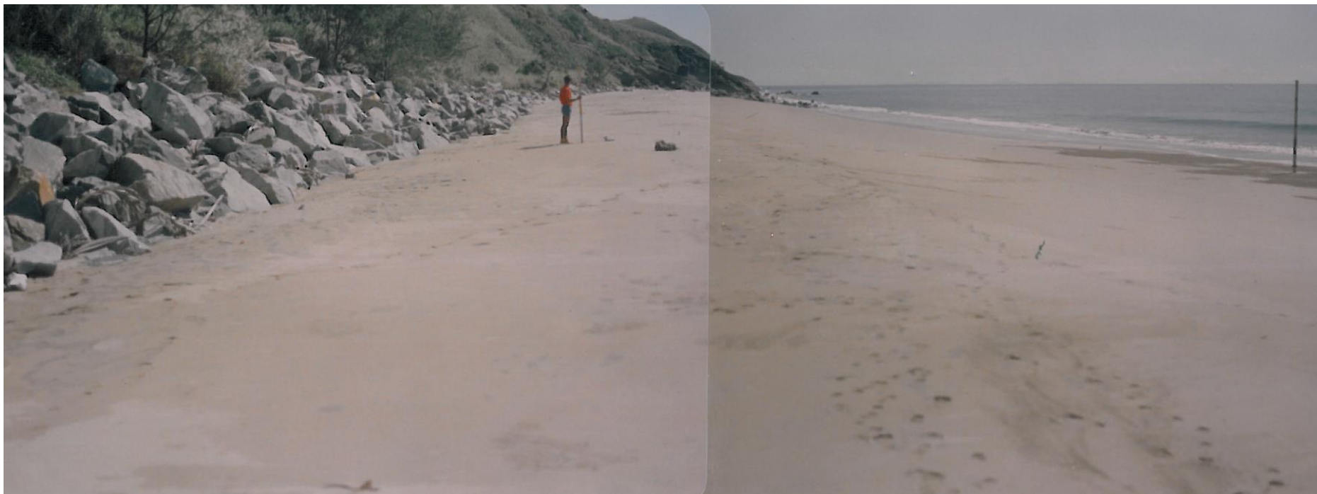
Figure 83 Blacks Beach looking North – May 1987
