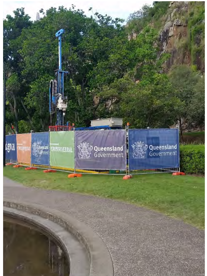
Drilling at the base of Kangaroo Point cliffs—the future tunnel will pass under this area.
