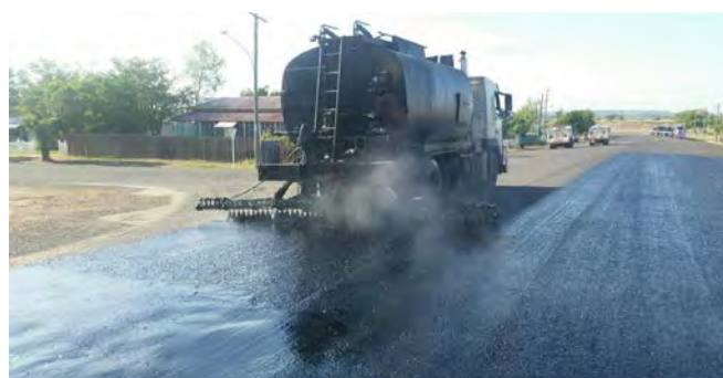
Rehabilitation work on Flinders Highway through Hughenden
