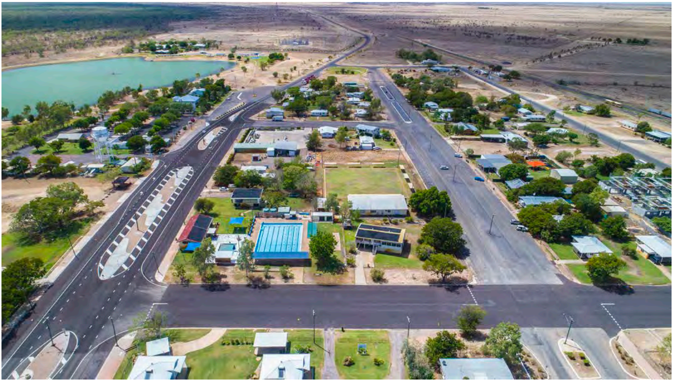
Completed works to Goldring Street, Richmond.
