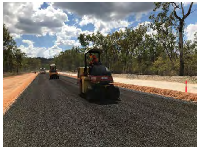
Sealing works at Ten Mile Creek
