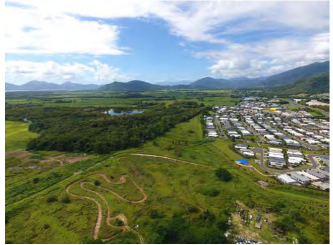
Looking south along the alignment of the future Smithfield Bypass Road, which passes around Cattana Wetlands.
