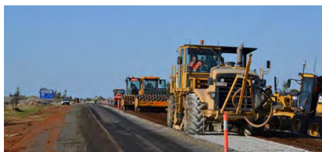
Pavement rehabilitation and overlay, extension of road width and sealing on the Landsborough Highway between Augathella and Tambo.
