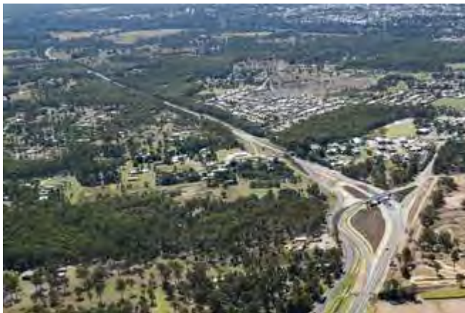
Looking north over the Tinana interchange on the Bruce Highway. Image provided courtesy of Georgiou Group.
