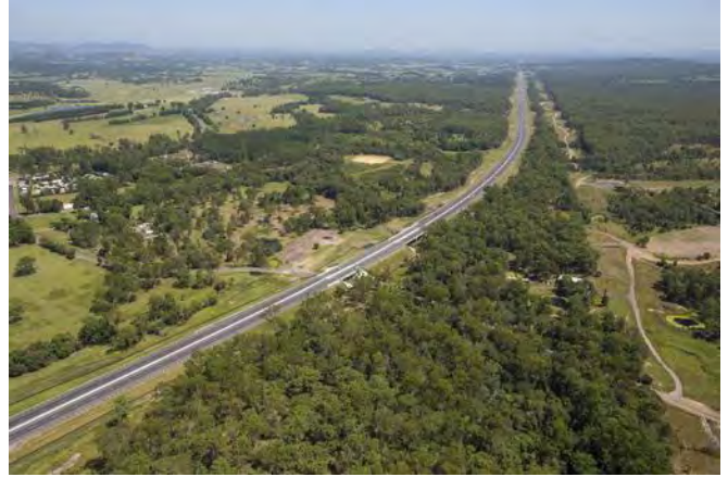
Cooroy to Curra (Section C) from Tandar Road overpass looking north.
