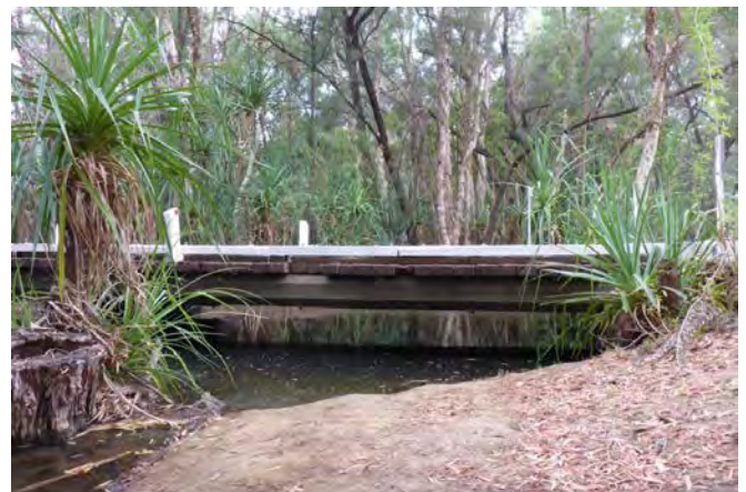
Beames Brook (Julia Creek – Burketown Road) original 1950s single lane timber bridge.
