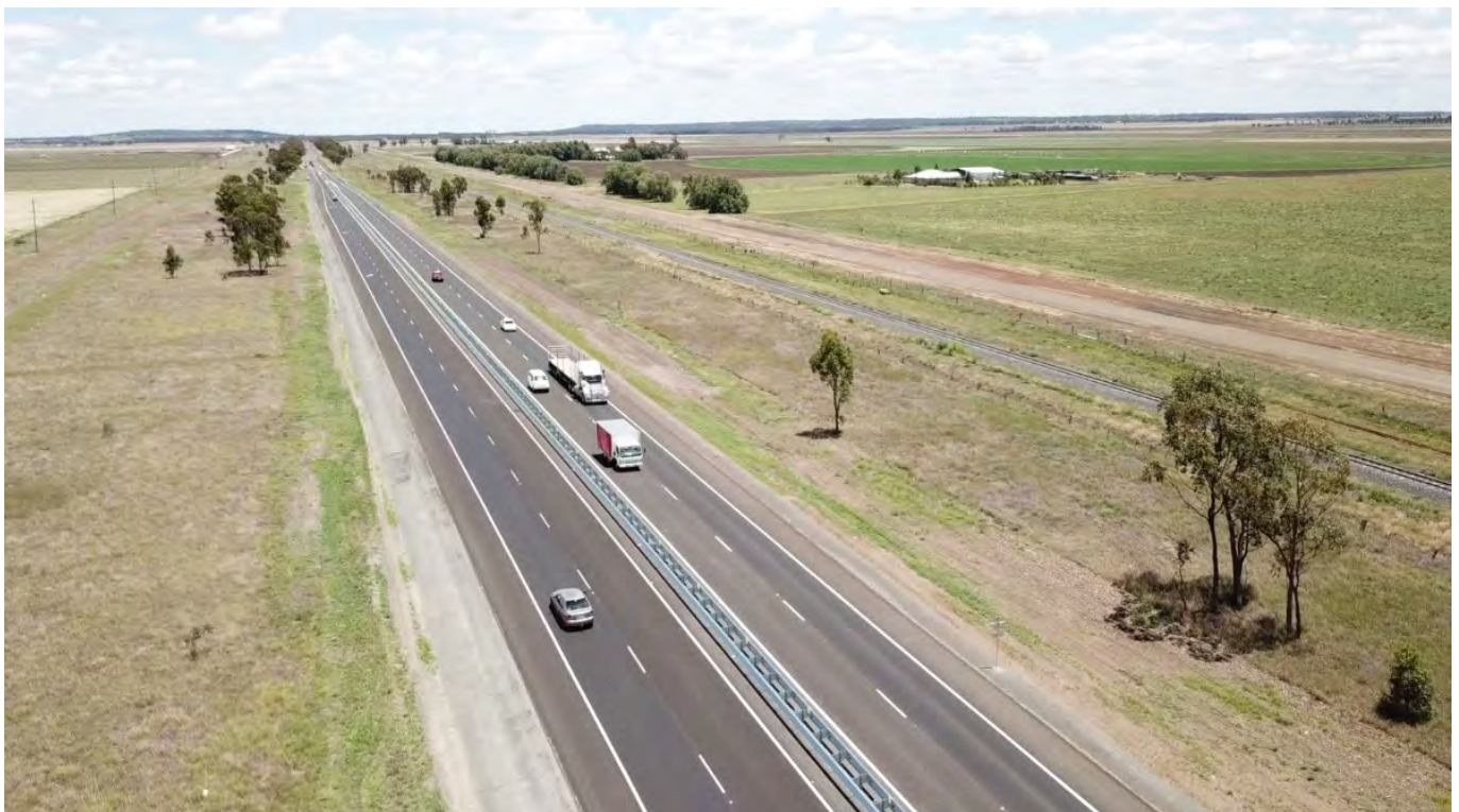
Opposing westbound and eastbound overtaking lanes, as part of the Oakey to Dalby Overtaking Lanes project.
