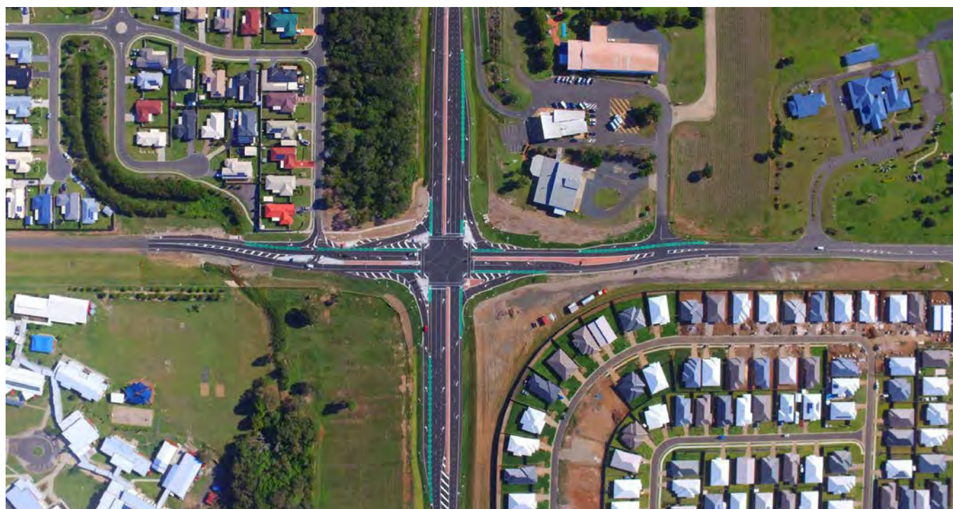
Aerial photo of upgraded Urraween Road intersection.
