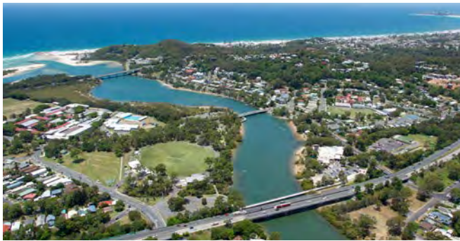
Pacific Motorway Currumbin Creek Bridge.
