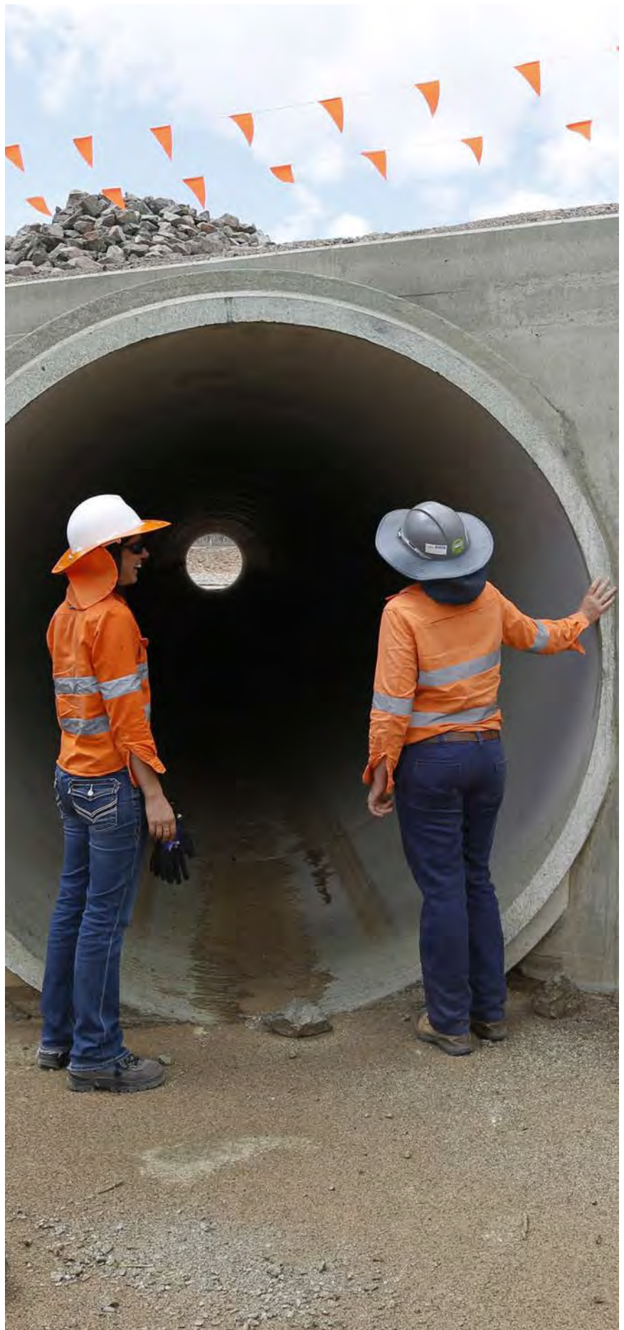
TMR staff inspecting construction
