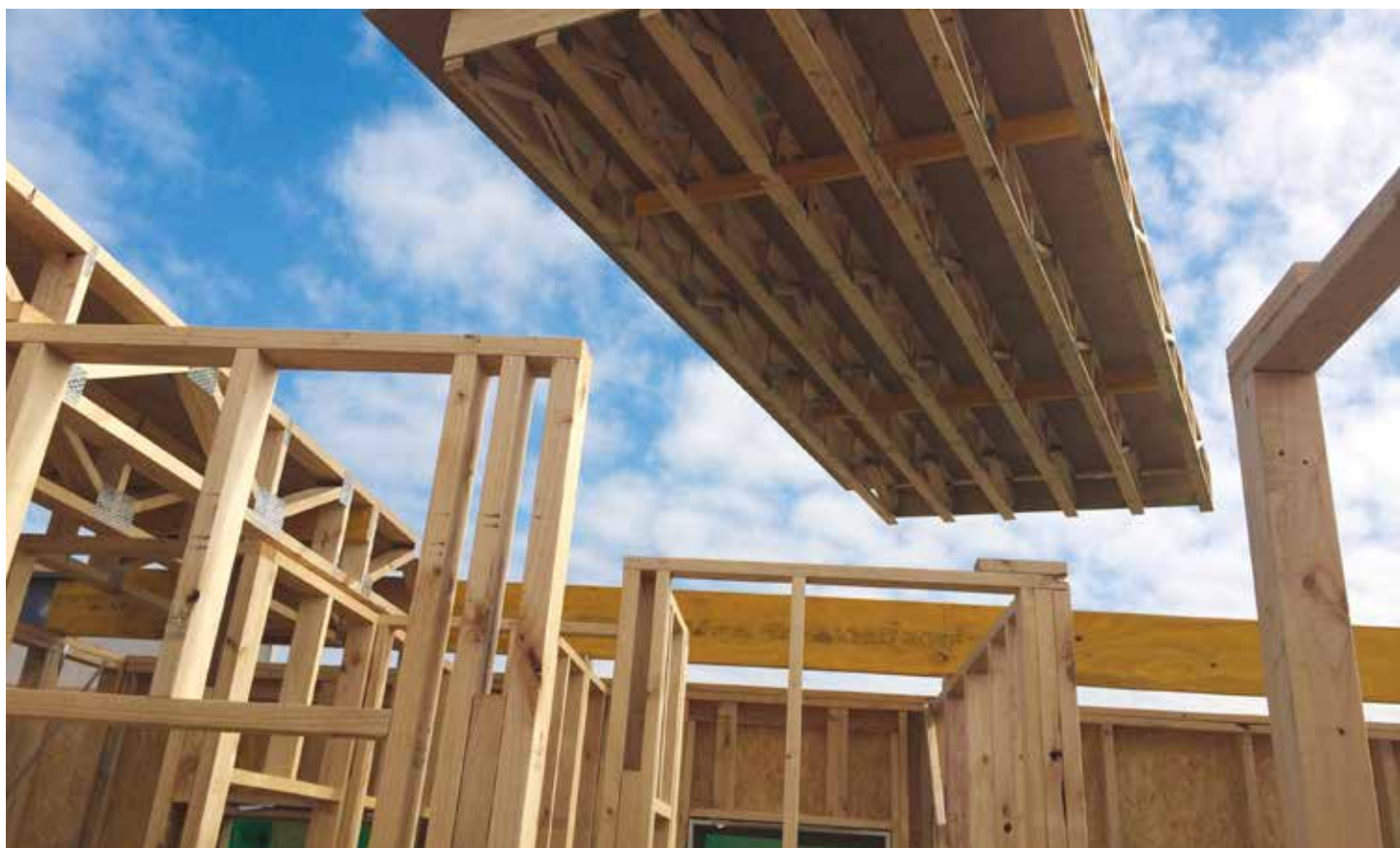
Prefabricated flooring system used in housing construction. Source: Pryda
