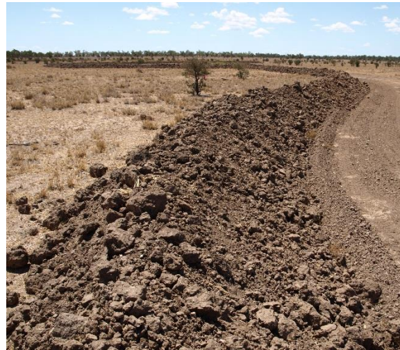
Photos of Illamahta gully site, showing a portion of the gully, contour bank and appropriate area to spread water from end of contour.
