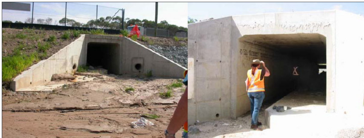
Figure 4. Example of multiuse culverts showing ledge design. Note. Culverts in figure are larger dimensions than what is being proposed (Source: Goosem 2005).
