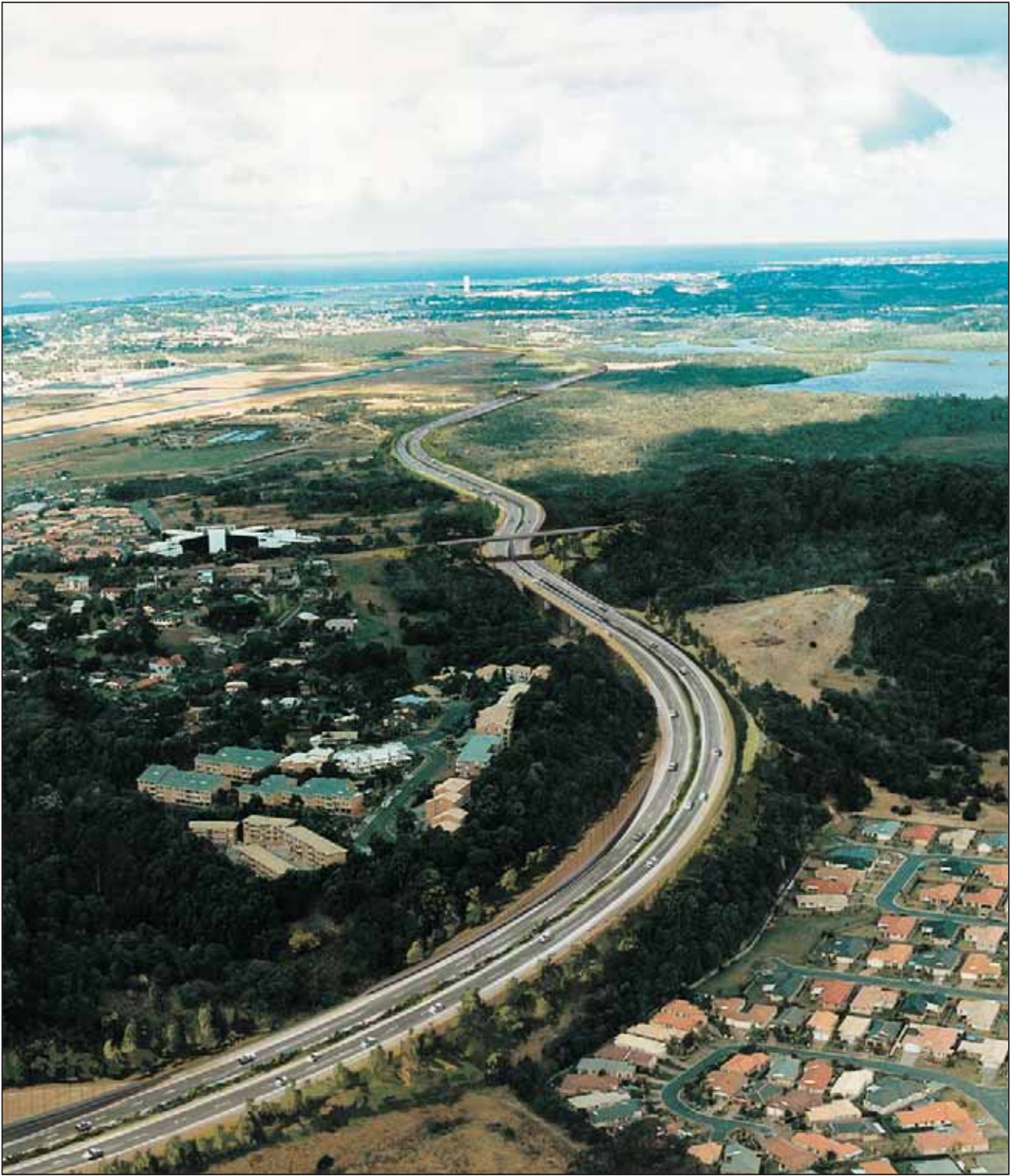
Figure 1.2b The Tugun Bypass Looking South
