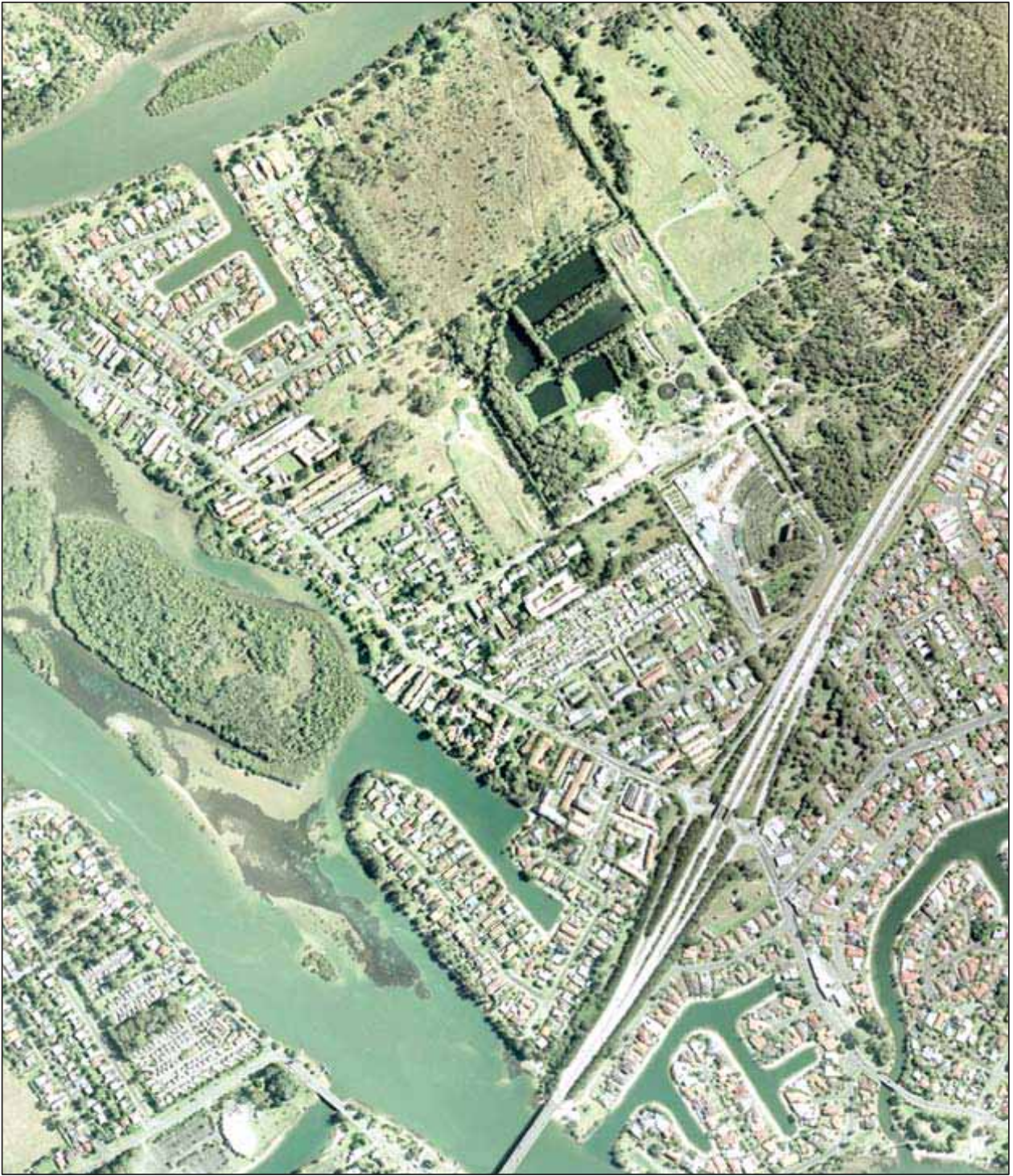
Figure 1.2a Stewart Road Interchange Looking Towards Tugun
