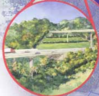
Hidden Valley Bridge
