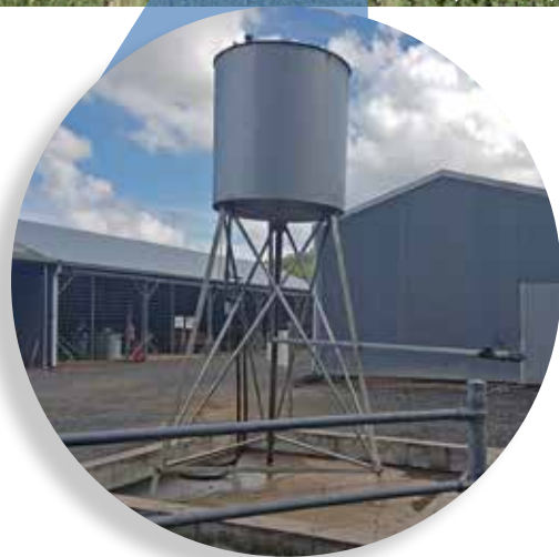
Figure 8: Fuel tank located on the edge of the farming zone
