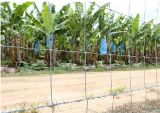
Figure 41: Hinge joint mesh fencing
