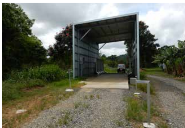
Figure 27: Spray grids can be suitable to disinfect low-risk vehicles that need to access your packing shed via your separation zone
