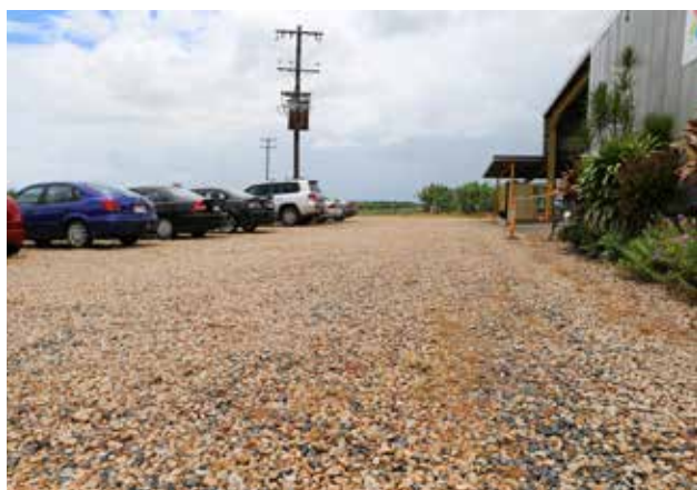
Figure 4: Surfaced exclusion zone
