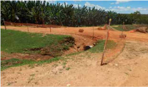
Figure 38: Example of earthworks and drains directing water away from a production area
