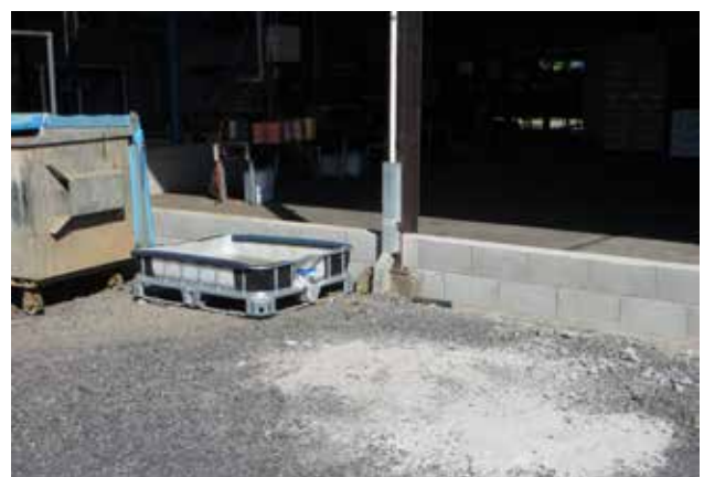
Figure 37: Barriers such as brick walls are also a good way to limit movement between zones
