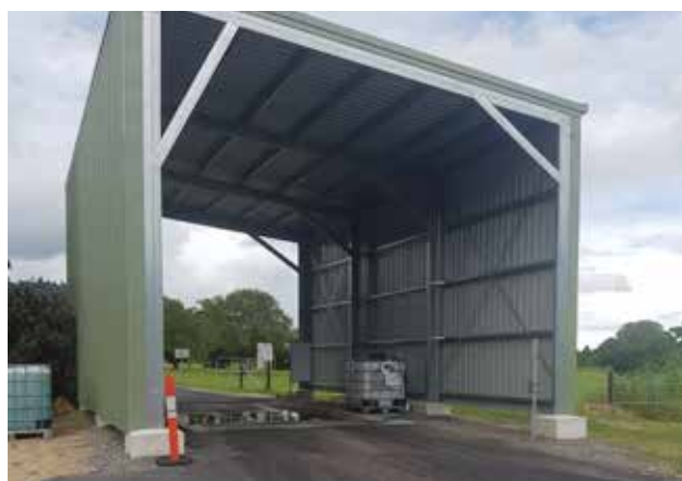
Figure 32: Vehicle dips located in high rainfall areas should have a roof over them
