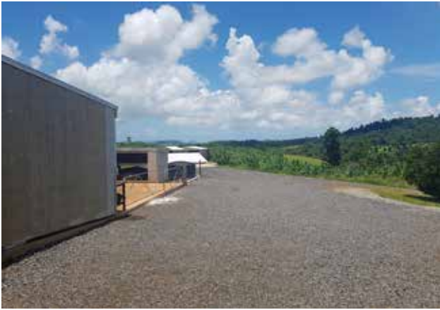
Figure 22: Hard-surface access road with fencing to minimise risk of accidental movement
