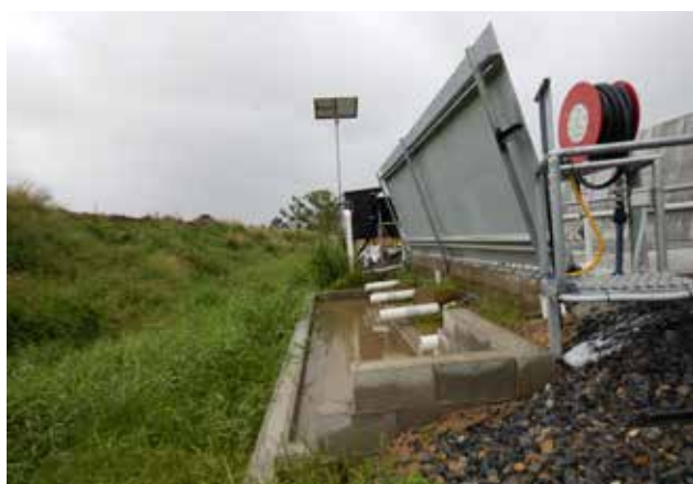
Figure 29: An example of waste water being contained
