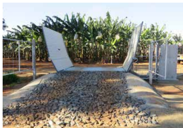
Figure 28: An example of gravel at the approach and exit of a spray grid
