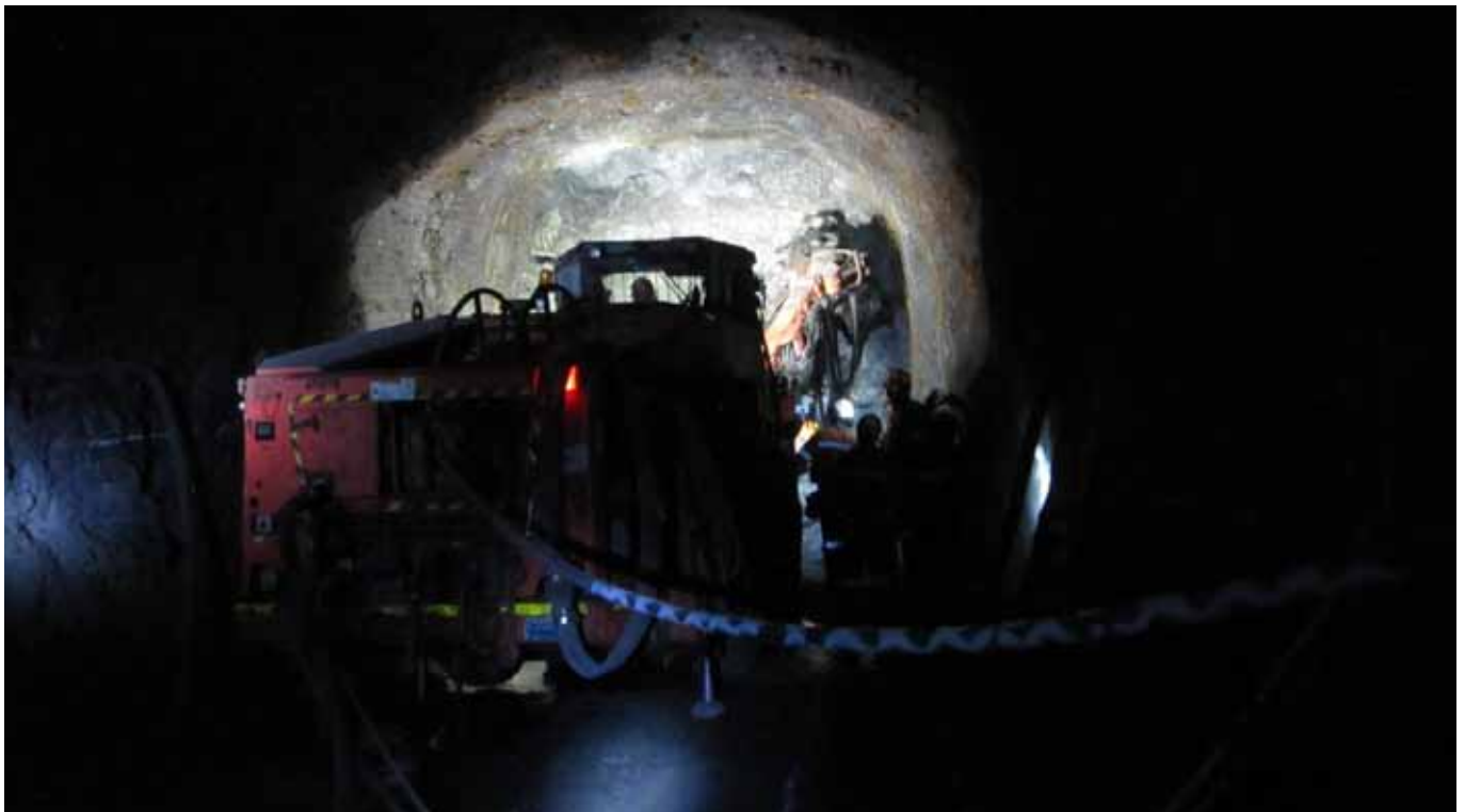
Twin boom development jumbo drilling out a face for charging Photo: DNRM
