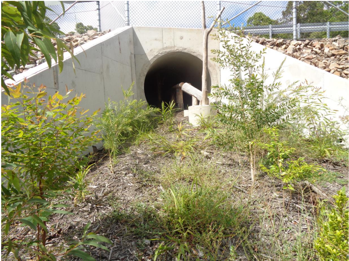
Figure 5. Completed Northern Fauna passage
