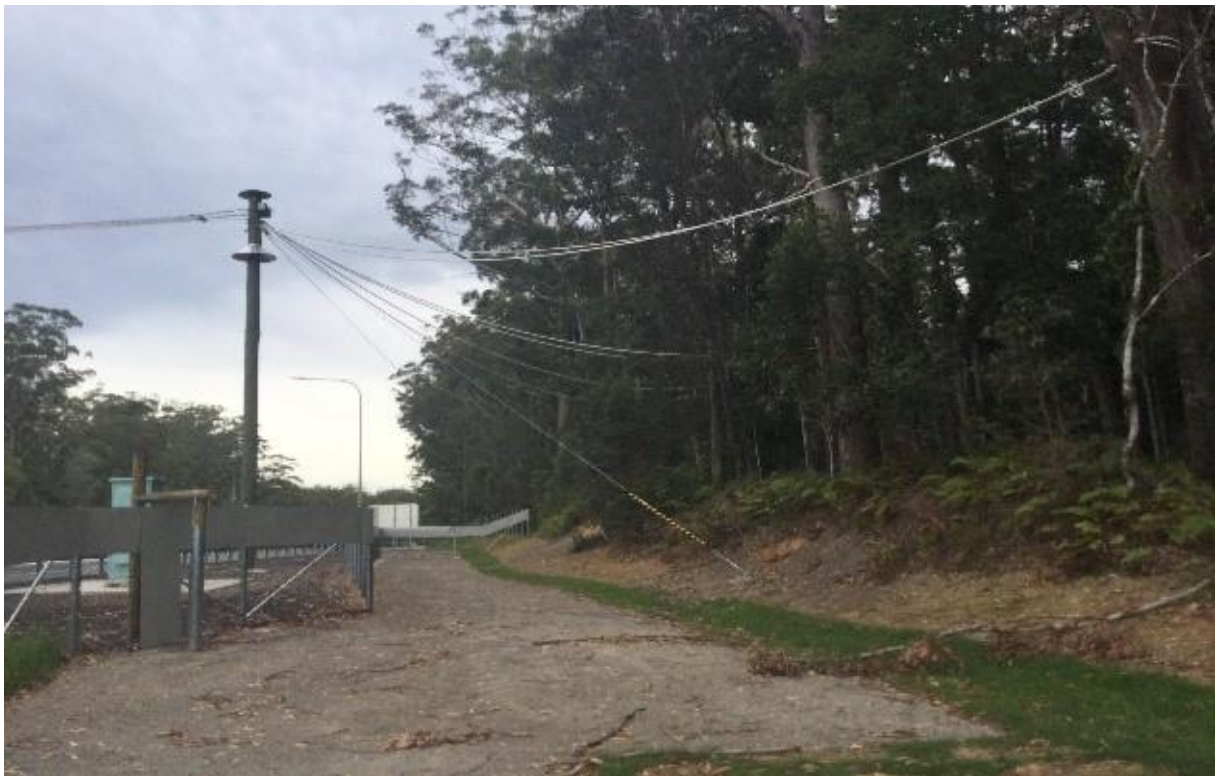
Figure 11. Rope Bridge across Steve Irwin Way
