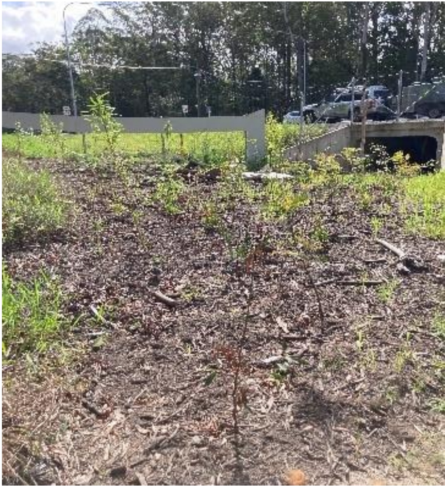
Figure 2. Completed Steve Irwin Way Fauna passage
