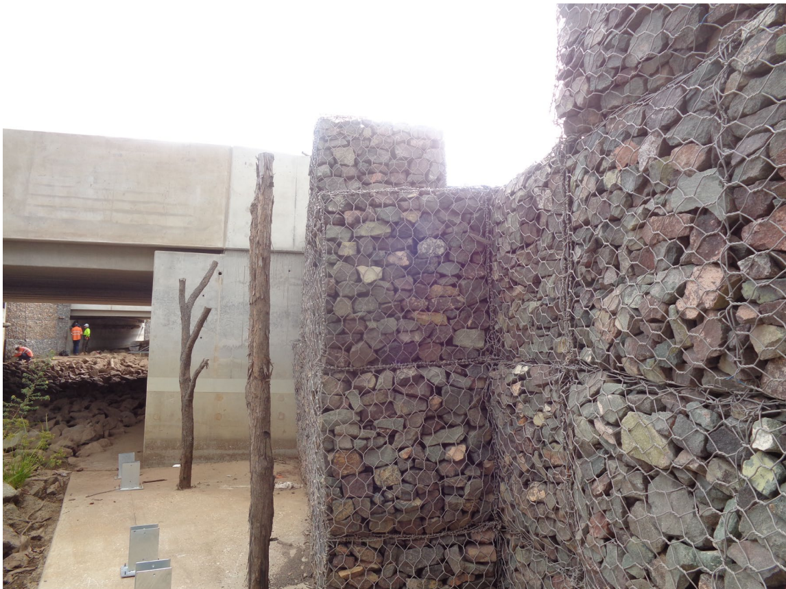
Figure 4. Fauna structures being installed on the southern side of Sippy Creek
