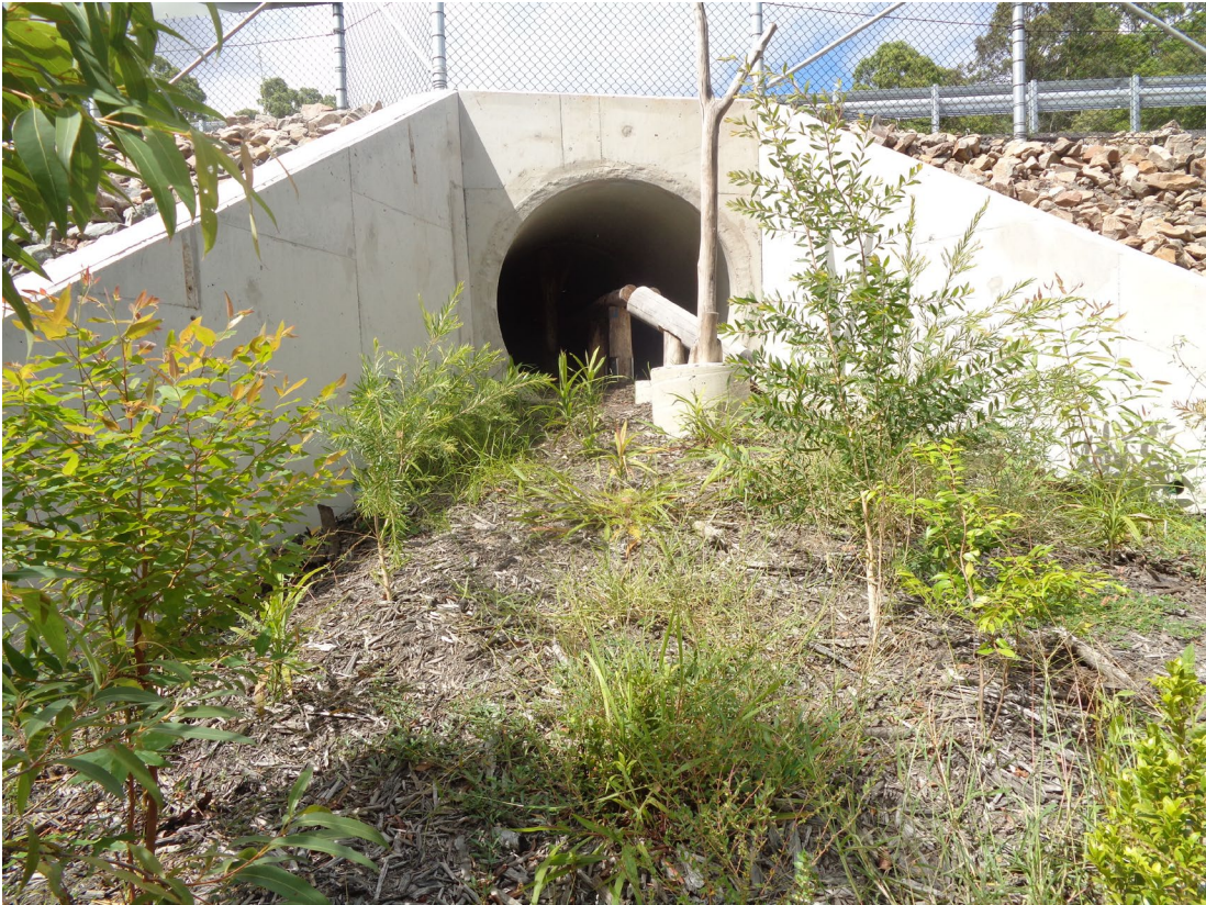
Figure 2. Completed Northern Fauna passage (CU-17-03)
