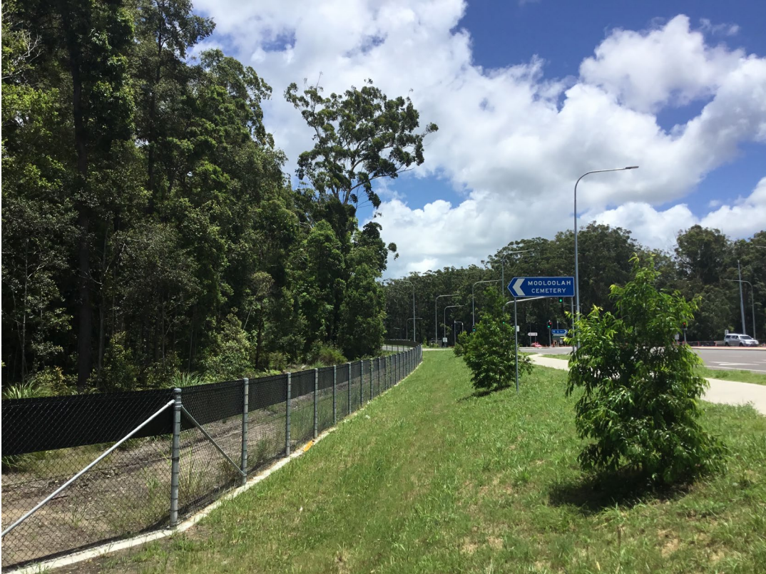
Figure 1. Permanent fauna fence adjacent to Mooloolah Cemetery
