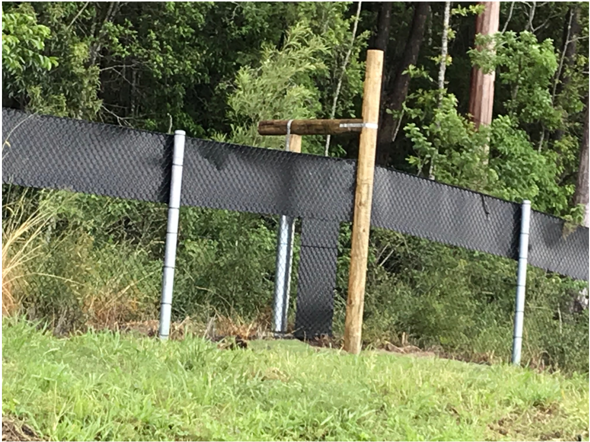
Figure 3. Koala escape pole along Wilson Road
